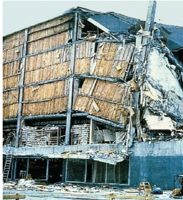
Penney's store, Anchorage, Alaska, earthquake, 1964. Left: Damage to the store: Right: Second-floor plan, showing unbalanced perimeter resistance
