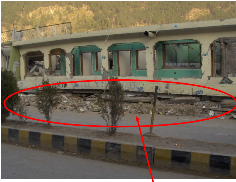
Lower story columns were collapsed in a hotel at Balakot, 2005 Kashmir earthquake
