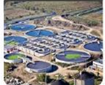
Water treatment, Waste Management
