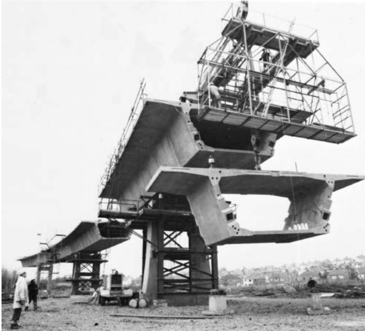
Posttensioned segmental precast concrete for East Moors Viaduct, Lanbury Way, Cardiff, South Wales. (Courtesy of Cement and Concrete Association.)
