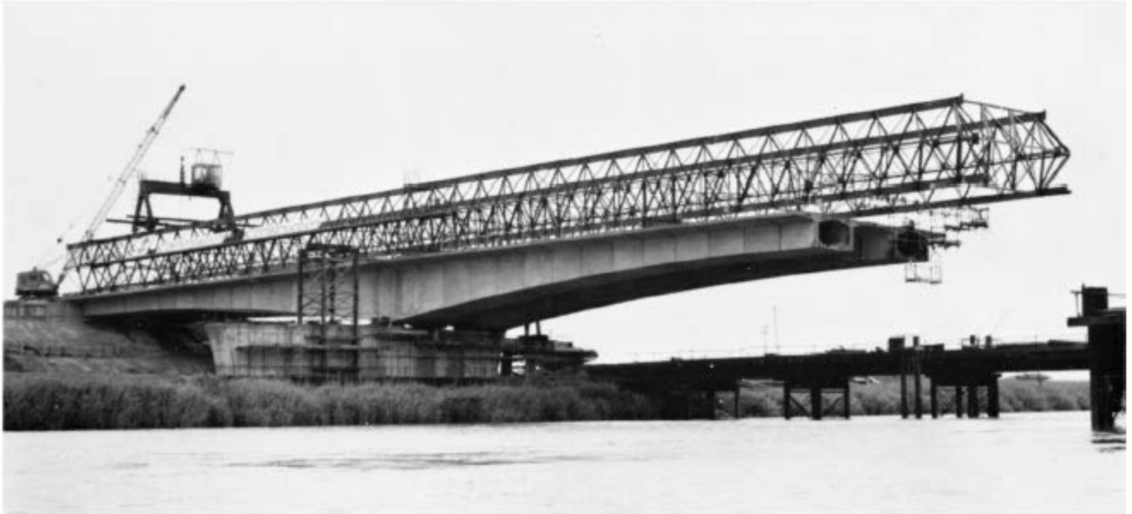
Prestressed concrete segmental bridge over the River Trent near Scunthorpe, Lincolnshire, England. (Courtesy of Cement and Concrete Association.)
