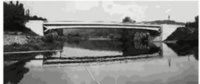
Fig. 4. Luzancy Bridge across the Marne River, France (1940). This elegant bridge (designed and built by Freyssinet) is the largest bridge in the world built of prestressed segmental construction.
