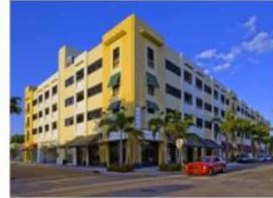
City of South Miami Municipal Parking Structure (Miami, FL)
