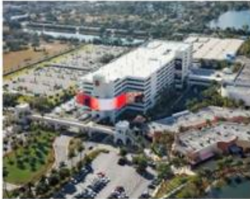
Seminole Hard Rock Hotel and Parking Structure (Hollywood, FL)
