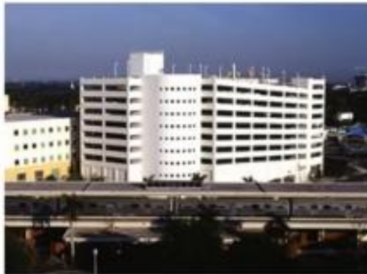
Miami Dade Water and Sewer Parking Structure (Miami, FL)
