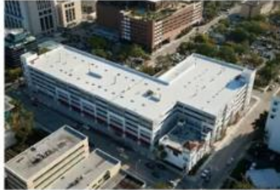
Broward County Courthouse Parking Structure (Fort Lauderdale, FL)
