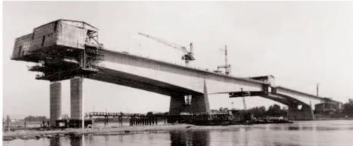
Fig. 7. Bendorf Bridge over the River Rhine, Germany (1962). (Designed by Ulrich Finsterwalder.)
