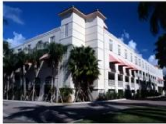
Turnberry Isles Country Club Parking Structure (Aventura, FL)
