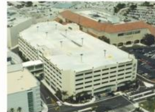
Open for Business (11 weeks after beginning of construction)
