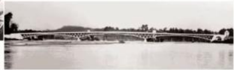
Fig. 1. Le Vieux Bridge across the Allier River, France (1910-1913). Spans were 222 - 238 - 223 ft (67.3 - 72 - 67.5 m). This bridge incorporated the first use of thrust by jacks at midspan for decreasing and also compensating for concrete creep and shrinkage. (Designed and built by Eugene Freyssinet.)
