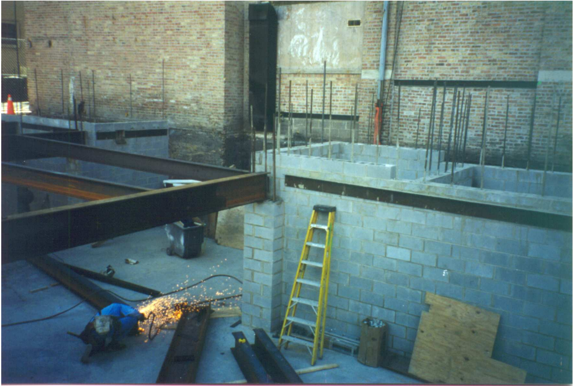
Welding steel beams at a construction site.
