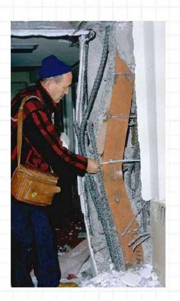
Buckling in a Composite column
