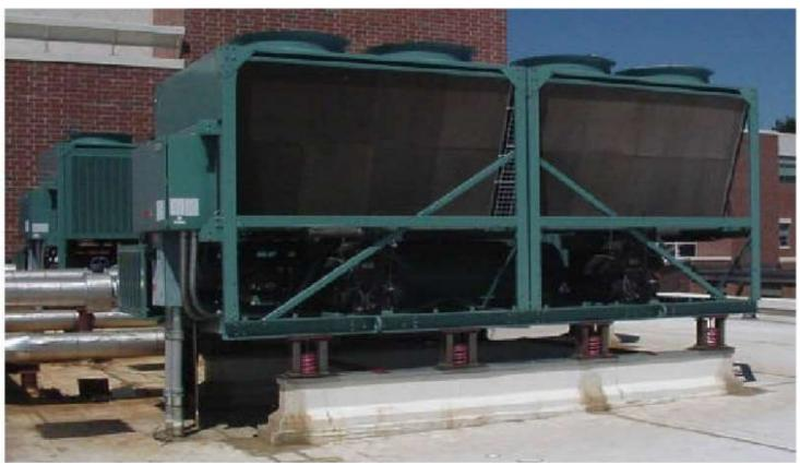
A reciprocating air conditioning compressor and chiller mounted on a flexible roof, Note the straight conduit on the left of which bypasses the isolators and directly transmit vibration into the roof **Prepared By: Engr. Khurshid Alam**
