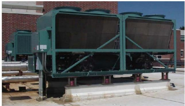
A reciprocating air conditioning compressor and chiller mounted on a flexible roof, Note the straight conduit on the left of which bypasses the isolators and directly transmit vibration into the roof
