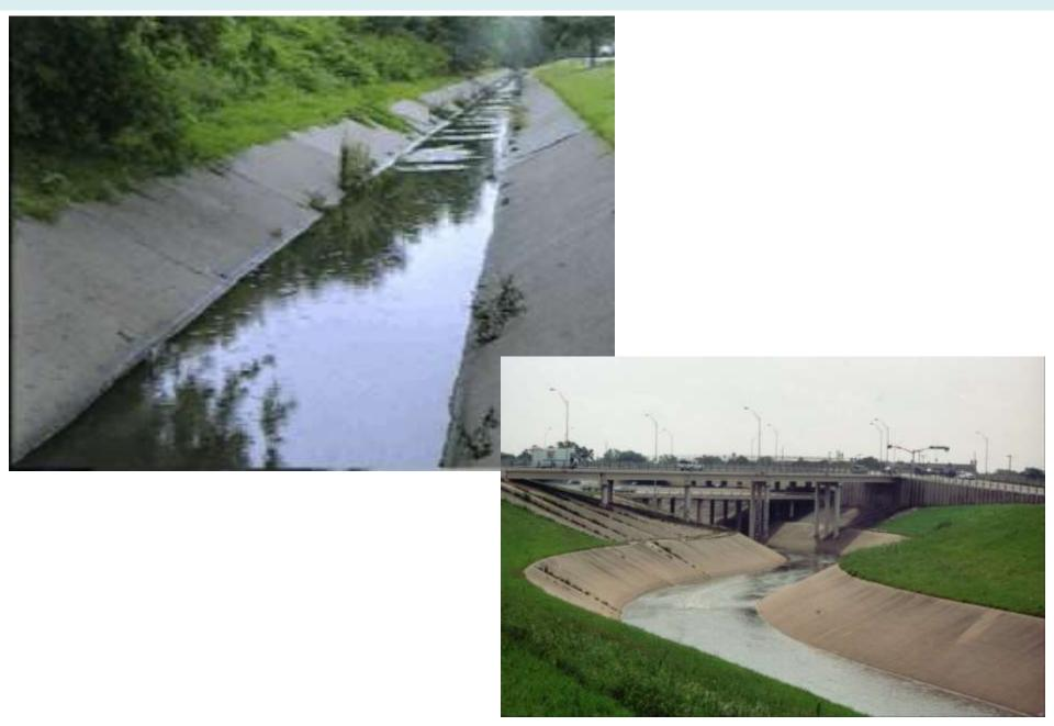
Based on their shape, an open channel can be prismatic or non-prismatic:
