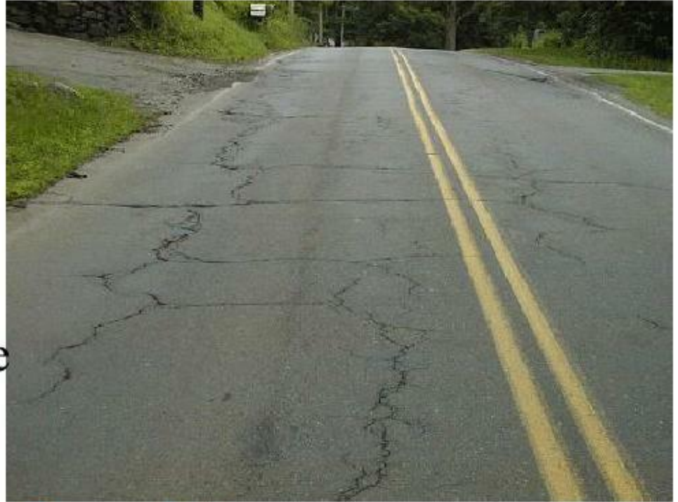
Block Cracking
