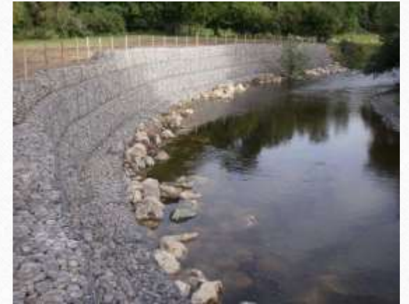
Gabion wall Flood Protection
