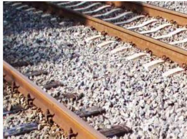
Railway Track Construction
