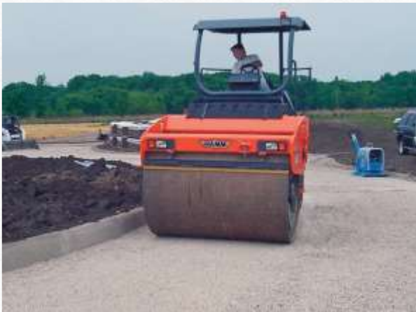
Road Base, sub-Base and wearing coarse Construction
