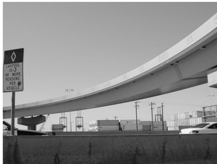
Box Girder Bridge
