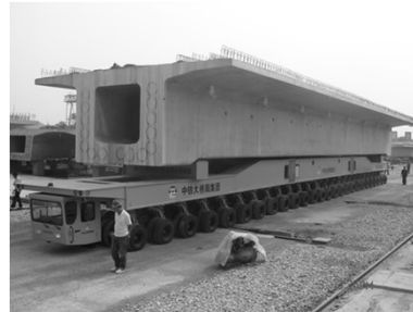
Concrete Box Girder Bridge
