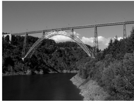
Steel Truss Arch
