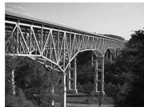
Steel Deck Truss Bridge
