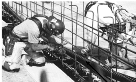
Post tensioning under progress
