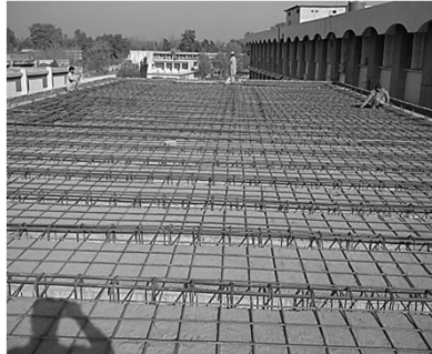
Slab Reinforcement
