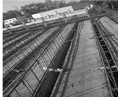
Beam Reinforcement
