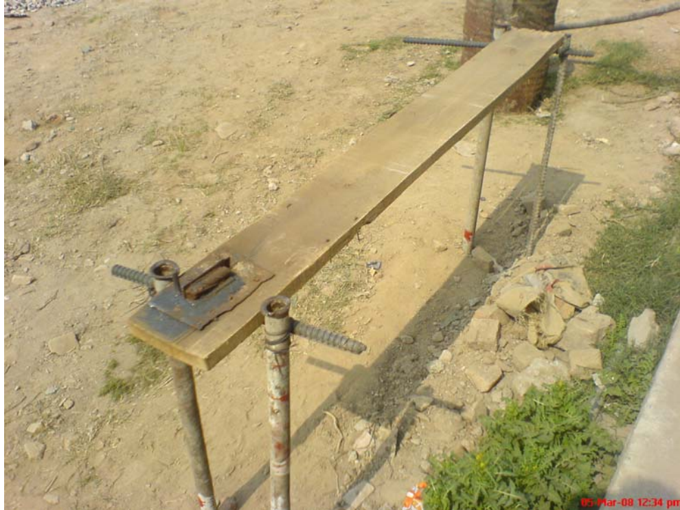
Figure 16: Local arrangement for bar bending.
