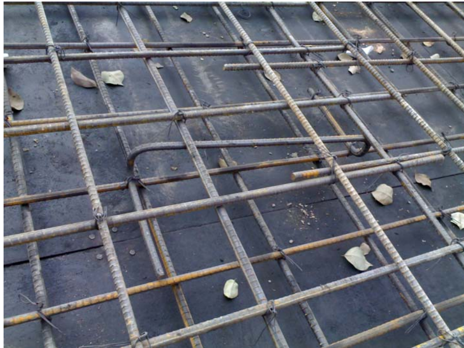
Figure 14: Supporting chairs for slab reinforcement.
