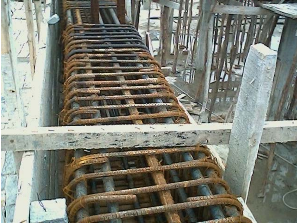
Figure 16: Flexure and shear reinforcement in a beam.
