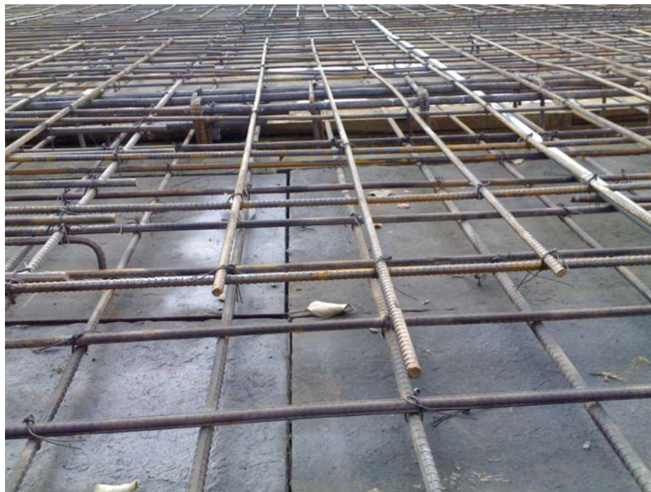
Figure 15: Reinforcement in slab.
