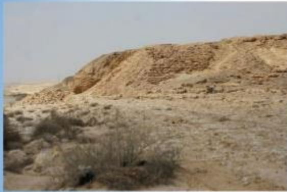
Sadd-el-Kafara Dam, Egypt 2800-2600 BC
