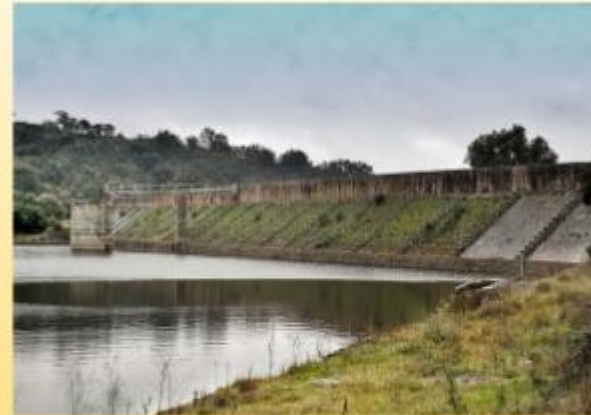
The Roman dam at Cornalvo, Spain has been in use for almost two millennia.
