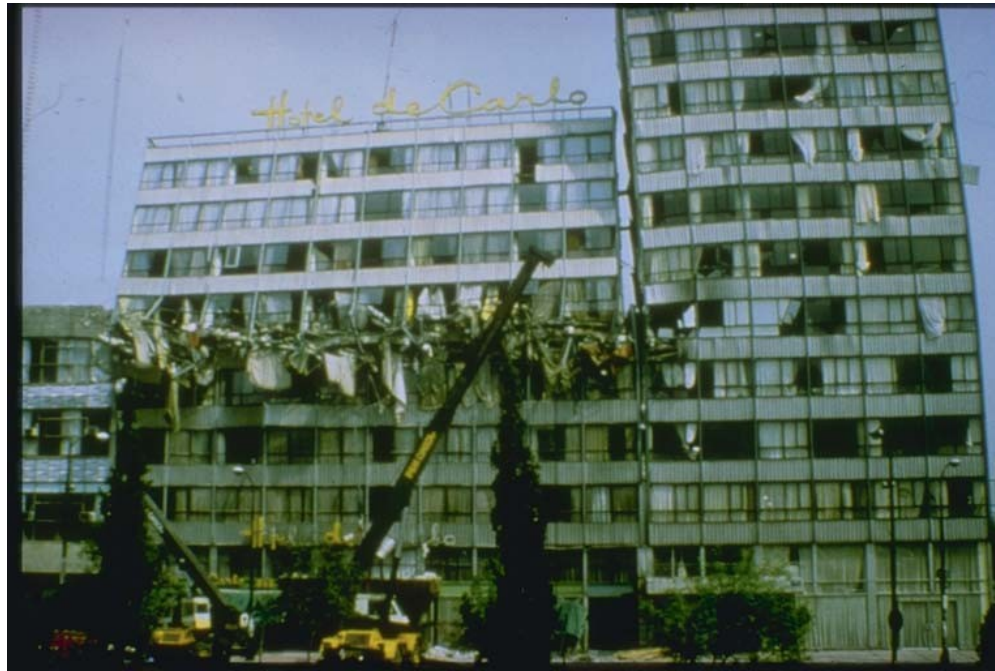
Pounding damage, Hotel de carlo, Mexico city, 1985 earthquake
