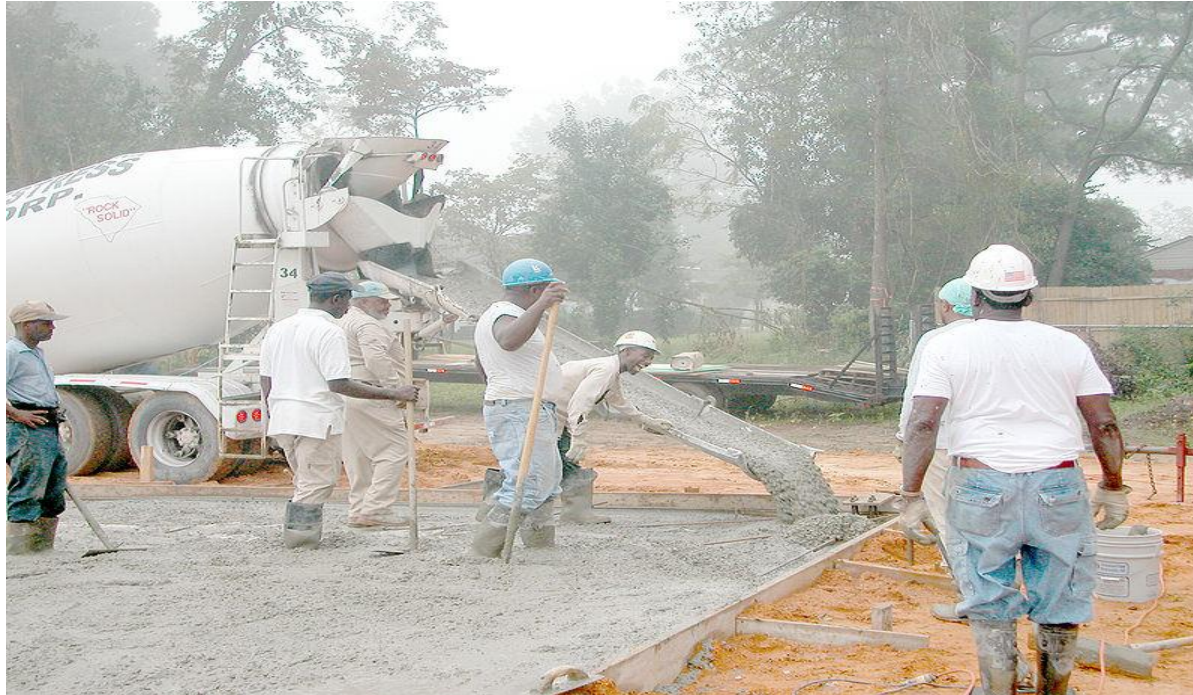
Pouring a concrete floor for a commercial building
