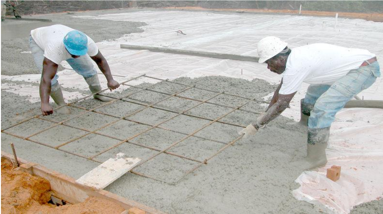
Installing rebar in a concrete floor during a pour
