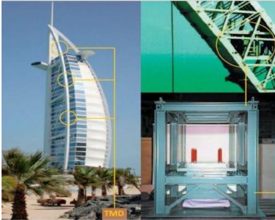
Tuned mass damper of Burj Al Arab
