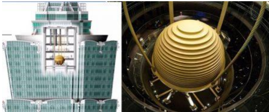
Tuned mass damper of Taipei structure
