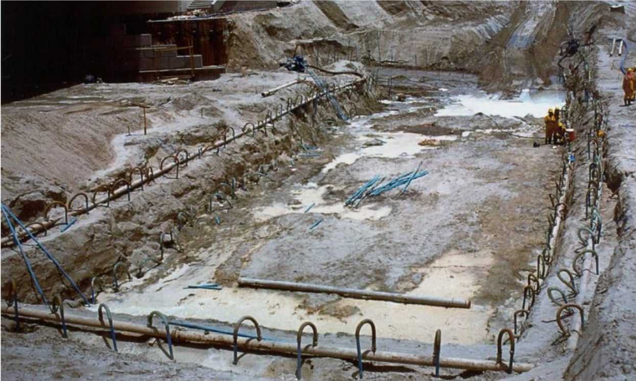
Well Point Dewatering
