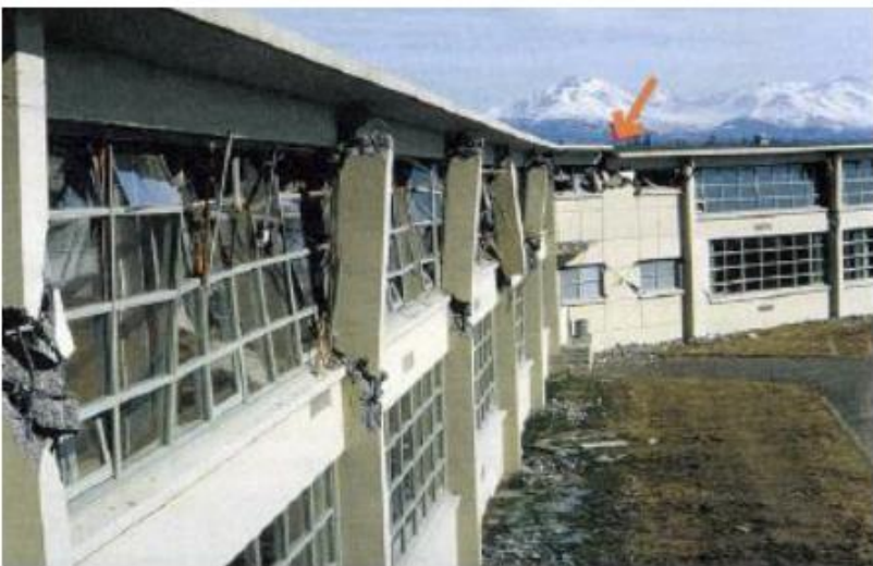
Figure 3 is the type of “Re-entrant corners”
