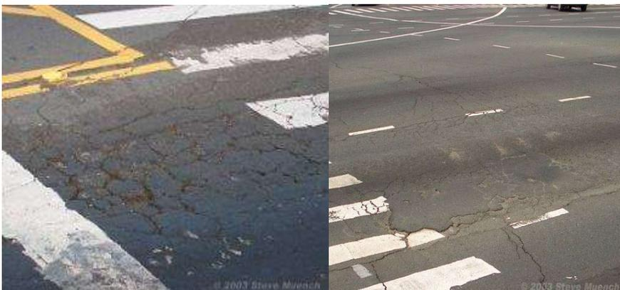
A series of interconnected cracks caused by fatigue failure of the HMA surface under repeated traffic loading. As the number and magnitude of loads becomes too great, longitudinal cracks begin to form (usually in the wheel paths). After repeated loading, these longitudinal cracks connect forming many-sided sharp-angled pieces that develop into a pattern resembling the back of an alligator or crocodile.
