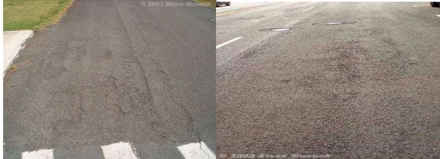
The progressive disintegration of an HMA layer from the surface downward as a result of the dislodgement of aggregate particles.
