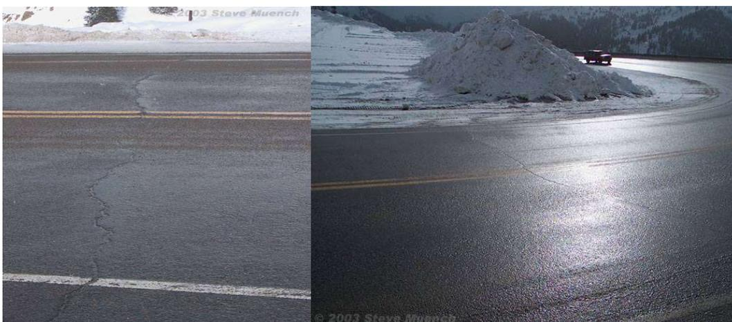
Cracks perpendicular to the pavement's centerline or laydown direction. Usually a type of thermal cracking.
