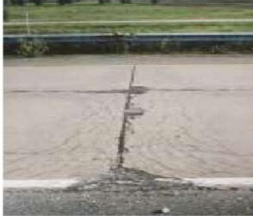
“D” cracking usually appears as a pattern of cracks running in the vicinity of and parallel to a joint or linear crack. It is caused by the concrete’s inability to withstand environmental factors such as freeze-thaw cycles because of variable expansive aggregates.
