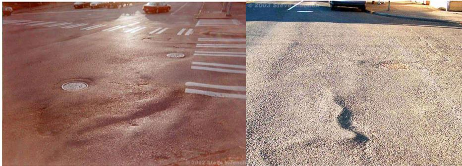
A form of plastic movement typified by ripples (corrugation) or an abrupt wave (shoving) across the pavement surface. The distortion is perpendicular to the traffic direction. Usually occurs at points where traffic starts and stops (corrugation) or areas where HMA abuts a rigid object (shoving).
