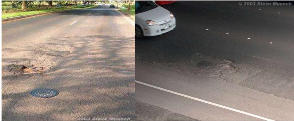
Small, bowl-shaped depressions in the pavement surface that penetrate all the way through the HMA layer down to the base course. They generally have sharp edges and vertical sides near the top of the hole. Potholes are most likely to occur on roads with thin HMA surfaces (1 to 2 inches) and seldom occur on roads with 4 inch or deeper HMA surfaces.
