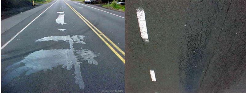
A film of asphalt binder on the pavement surface. It usually creates a shiny, glass-like reflecting surface that can become sticky when dry and slippery when wet. Loss of skid resistance when wet, unsightly
