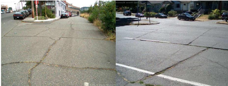
Vertical or horizontal movements in the pavement beneath an overlay cause this type of distress. These movements may be due to expansion and contraction caused by temperature and moisture changes or traffic loads. The cracks in asphalt overlays reflect the crack pattern in the underlying pavement.
