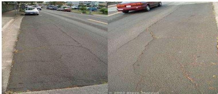
Shrinkage of the asphalt concrete and daily temperature cycling, which results in daily stress/strain cycling, causes block cracking. These are interconnected cracks that divide the pavement into approximately rectangular pieces. This type of distress usually indicates that the asphalt has hardened significantly.
