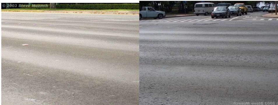
A rut is characterized by a surface depression in the wheel path. In many instances, ruts become noticeable only after a rainfall when the wheel paths fill with water. This type of distress is caused by a permanent deformation in any one of the pavement layers or subgrade, resulting from the consolidation or displacement of the materials due to traffic loads.
