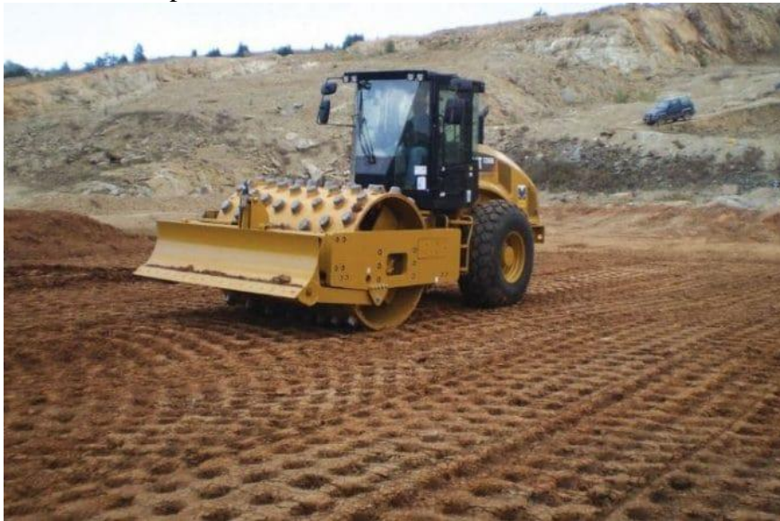
Fig 2: Compaction of Soil using Sheep-foot Roller
