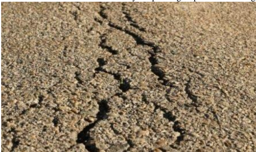
Fig 4: Shrinkage Cracks in Wet Compacted Soil
