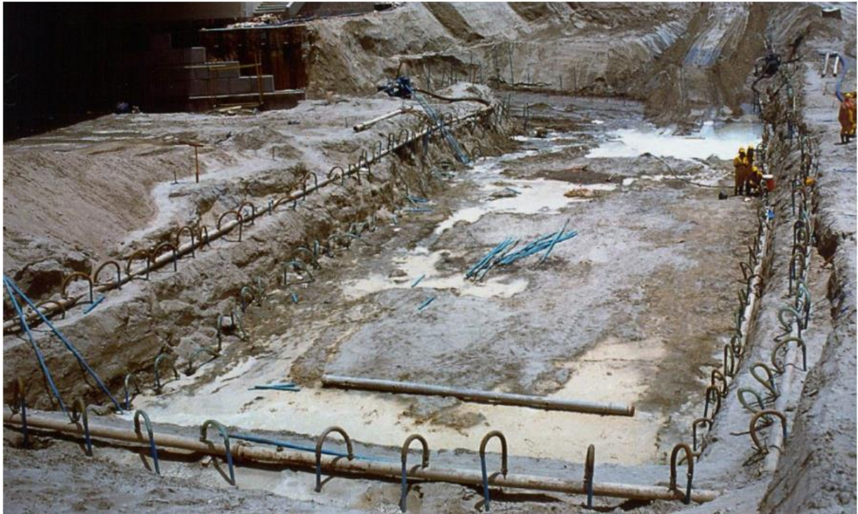
Well Point Dewatering
