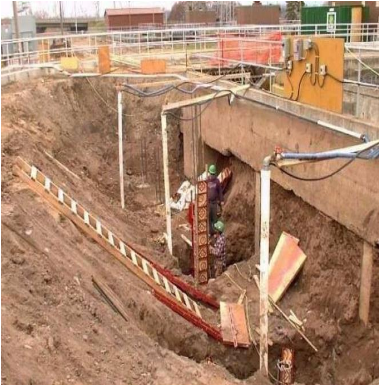
Deep Well Dewatering
