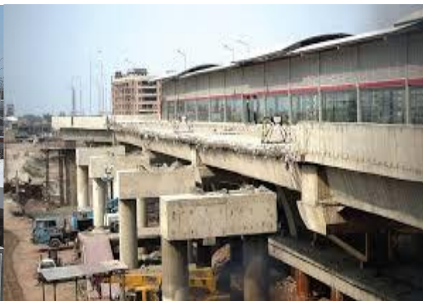
BRT station construction
