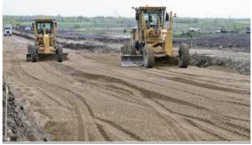
While the rolling progresses the entire surface of each layer shall be properly shaped and dressed with a motor grader, to attain a smooth surface free from ruts or ridges and having proper section and crown. Rolling shall continue until entire thickness of each layer is thoroughly and uniformly compacted to the specified density.
