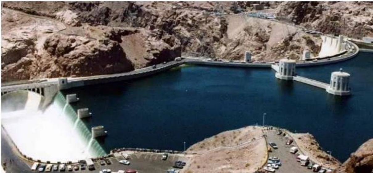
Figure: Side Channel Spillway
