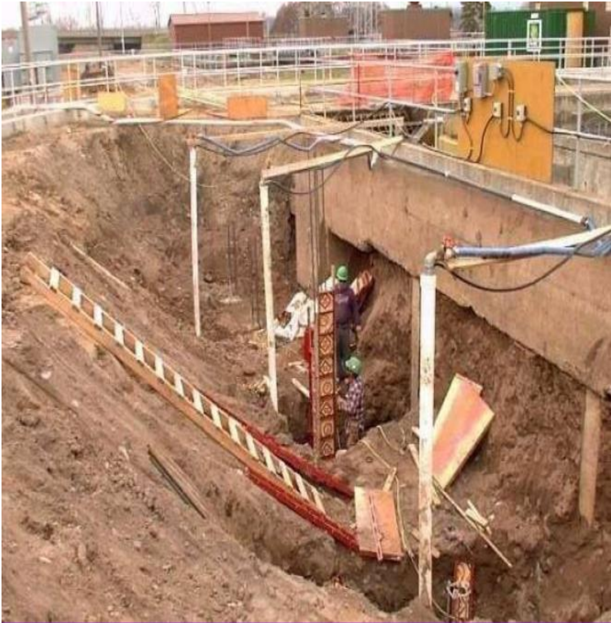
Deep Well Dewatering
