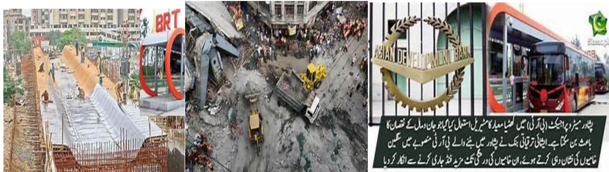
Figure 4: pictures show the corroded steel used in girders and other impure material
