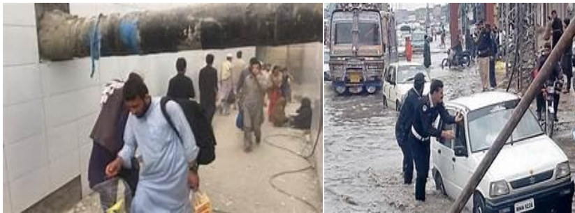
Figure 3: gas pipe in BRT underground rout and drainage supply disturb due to defective design
