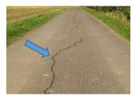
**1)** <u>Alligator (Fatigue) Cracking:</u> A series of interconnected cracks caused by fatigue failure of the HMA surface under repeated traffic loading. As the number and magnitude of loads becomes too great, longitudinal cracks begin to form (usually in the wheel paths). After repeated loading, these longitudinal cracks connect forming many-sided sharp-angled pieces that develop into a pattern resembling the back of an alligator or crocodile.
