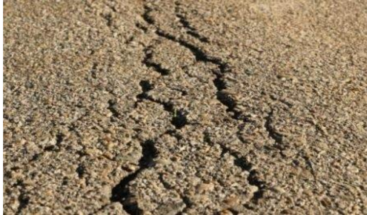
Fig 4: Shrinkage Cracks in Wet Compacted Soil
