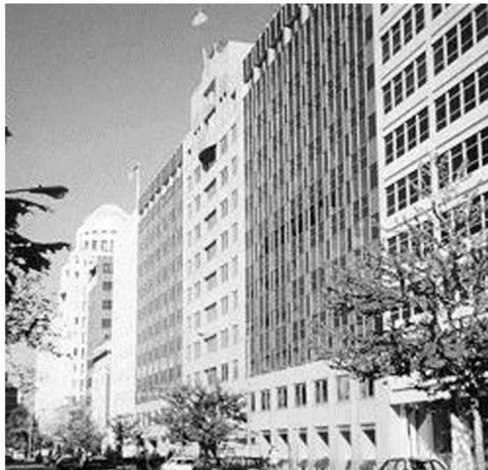
(above) The Matomac Building (second from right) at 1717 H Street N.W. served as headquarters for the U-2 project staff from February 1956 until March 1962, when the staff moved to CIA’s new headquarters at Langley, Virginia. CREDIT: Federation of American Scientists
