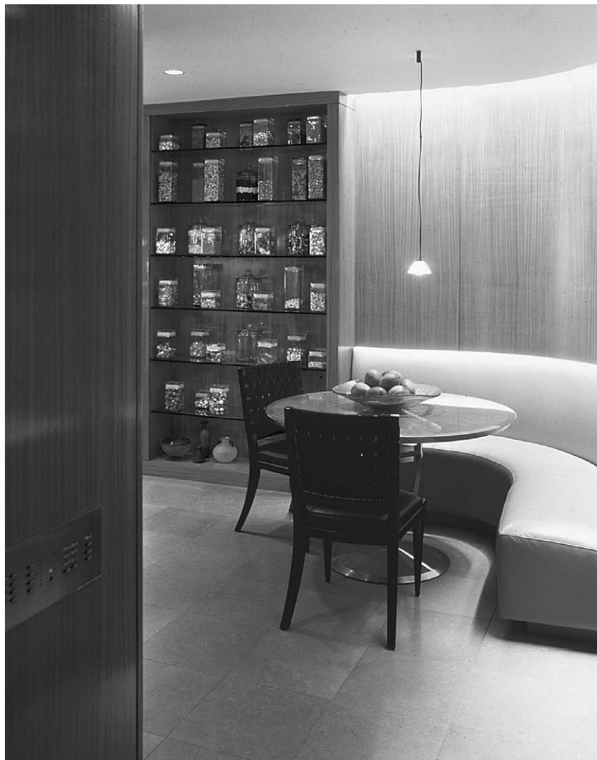
Figure 13.11 Continuous, linear, point-source wall wash.
