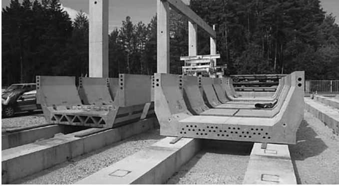
Fig. 7.41 Precast UHPC segments
