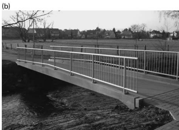
Fig. 7.25 First UHPC bridge in Germany: a) section, b) view of bridge after completion
