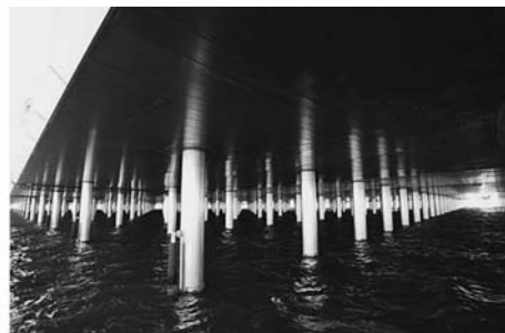
Fig. 7.61 Steel substructure with stainless steel jackets [Nippon Steel Corp.]
