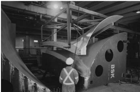
Fig. 7.56 Shell roofs to Shawnessy Light Rail Transit Station, Calgary, Canada (2004)
