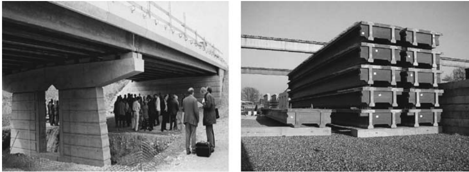
Fig. 7.3 Road bridge at Bourg-lès-Valence (left) assembled from prestressed double-T beams (right)
