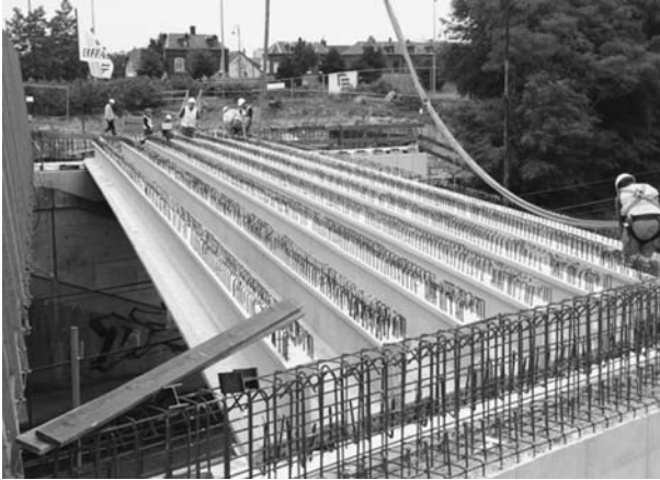
Fig. 7.6 Pont Pinel under construction
