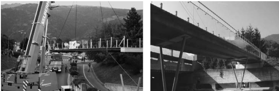
Fig. 7.39 Bridge for pedestrians/cyclists, Lienz
