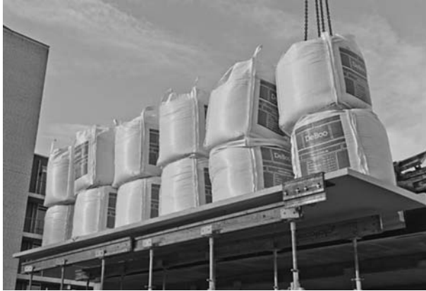
Fig. 7.55 Loading test on UHPC balcony (timber beams are for safety only)
