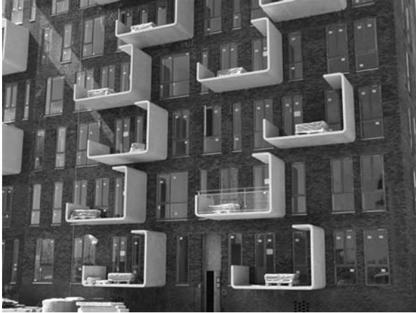
Fig. 7.53 White balconies made from fibre-reinforced UHPC (Hi-Con, Denmark [164])
