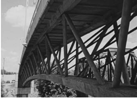
Fig. 7.1 Footbridge in Sherbrooke – the first ever bridge made from UHPC (1997)
