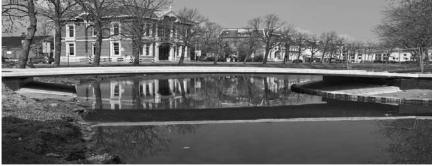
Fig. 7.44 Bridge made from UHPC for cyclists/pedestrians, Purmerend, The Netherlands (2008)
