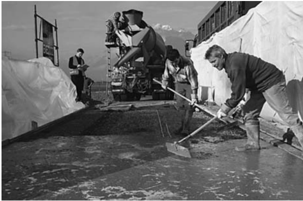
Fig. 7.43 Adding a layer of UHPC to a bridge deck (2004)
