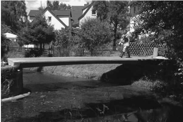
Fig. 7.26 Two further UHPC precast bridges over the River Nieste: a) section, b) view of one of the bridges
