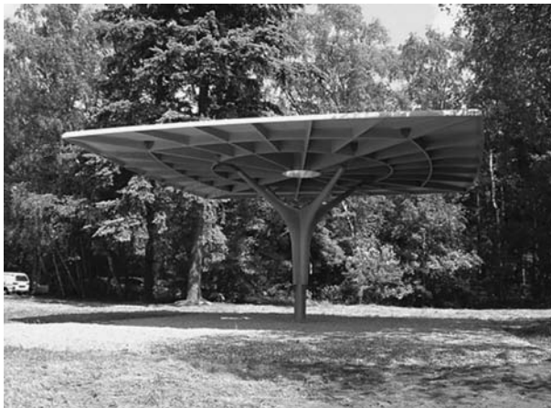
Fig. 7.57 UHPC canopy at entrance to 'De Zonnestraal' Hospital, Hilversum, The Netherlands (2005) [167]
