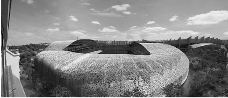
Fig. 7.65 Enclosing shell of precast UHPC elements for Jean Bouin Stadium, Paris [172]
