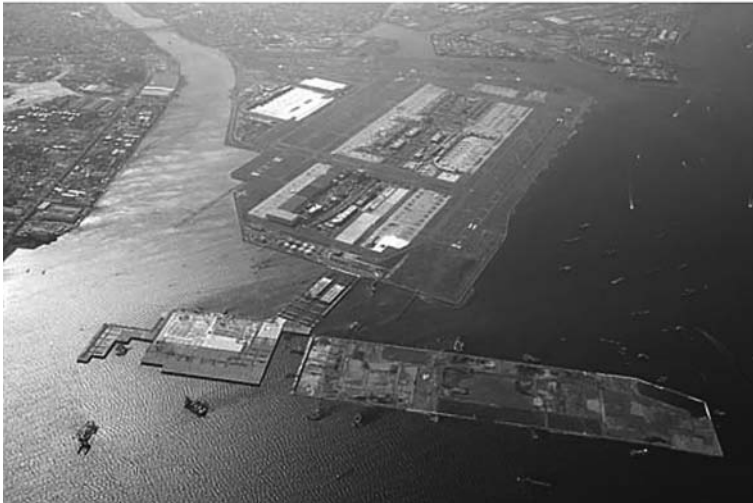
Fig. 7.60 New runway, Haneda Airport: a) computer image of design [170] for runway D, b) runway during construction. (Ductal®)
