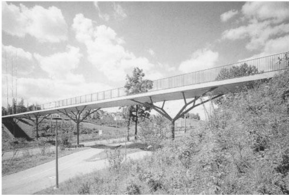
FIGURE 3.4 One of Jorg Schlaich's footbridges.
