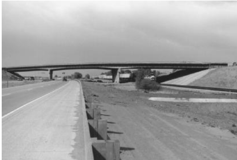
FIGURE 3.10 Buckley Road over I-76.
