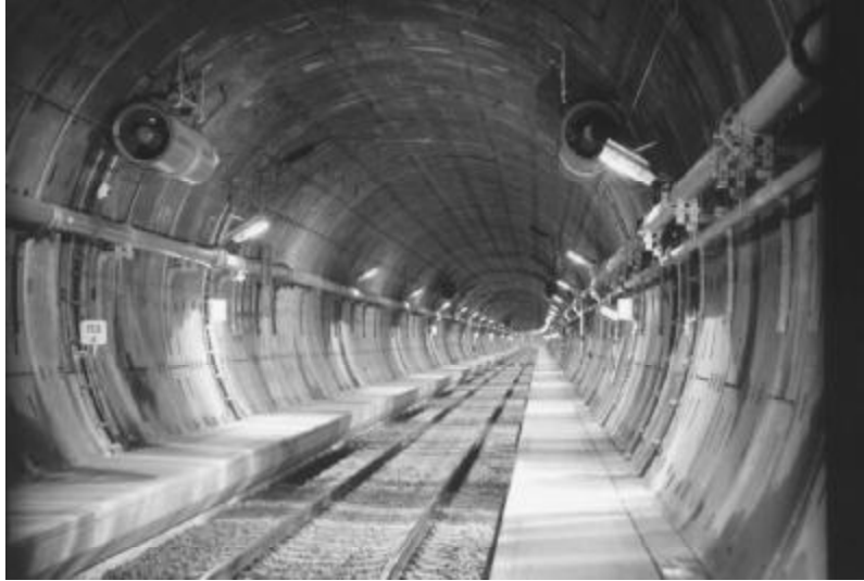
FIGURE 4.6 Storebælt East Tunnel.
