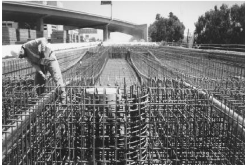
FIGURE 10.2 A post-tensioned box-girder bridge under construction.
