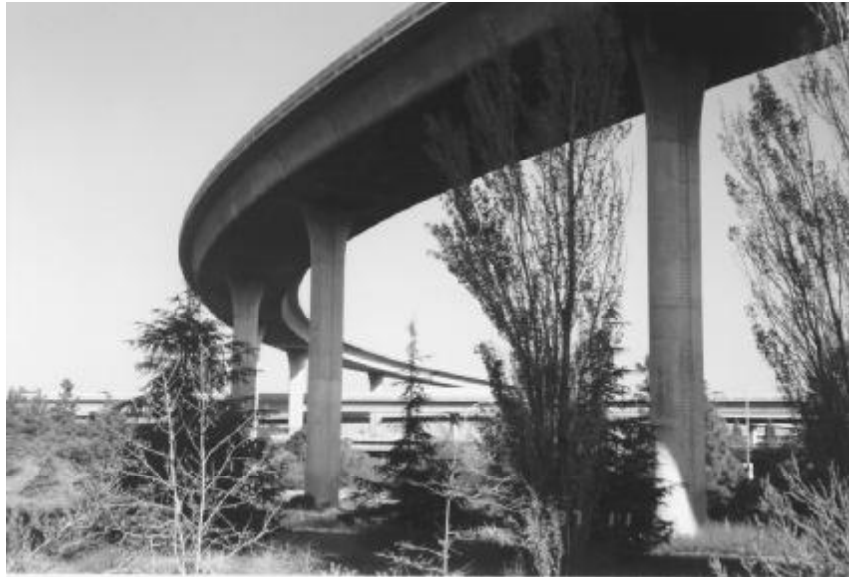
FIGURE 10.4 Prestressed box-girder bridge (I-280/110 Interchange, CA).
