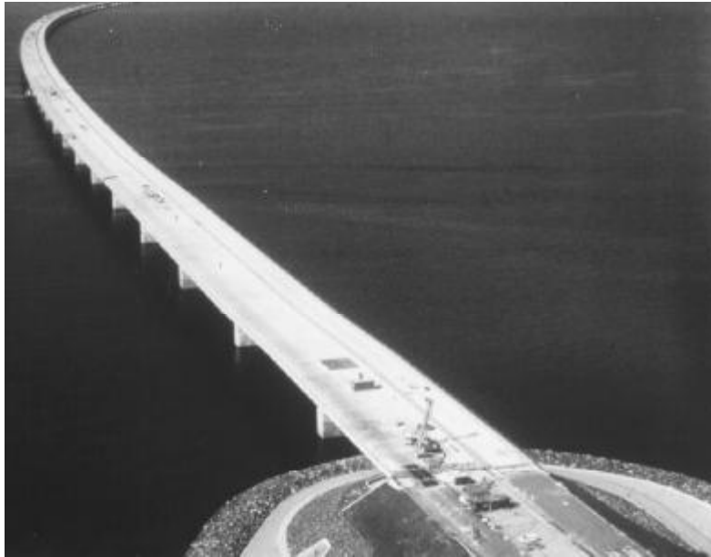
FIGURE 4.5 Storebælt West Bridge.
