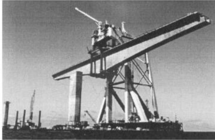
FIGURE 11.52 Confederation Bridge, Canada — floating crane.
