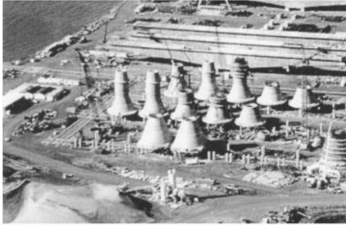
FIGURE 11.55 The Confederation Bridge, Canada — Prince Edward Island precasting yard.
