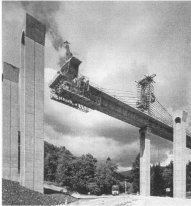
FIGURE 11.7 Fréburge Viaduct, France—erection with movable stay tower.
