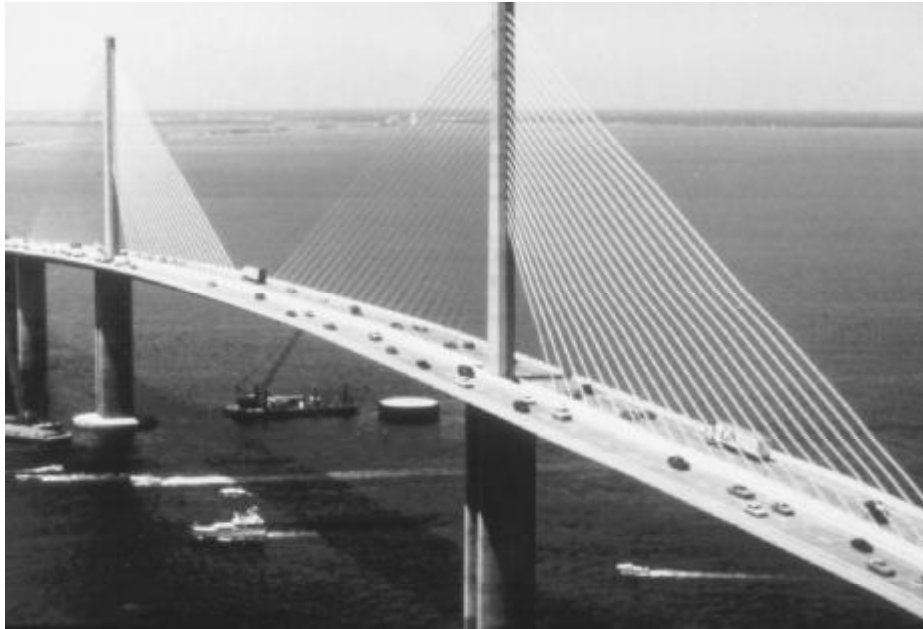
FIGURE 3.5 The Sunshine Skyway.
