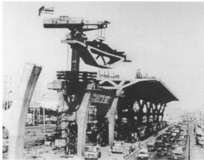
FIGURE 11.11 Bang Na Expressway, Thailand — launching of girder erection.
