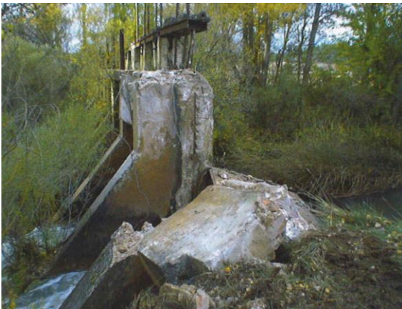
During the works
