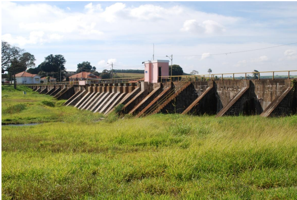
Fig. 2.15 – Barra Buttress Concrete dam, Brazil.
