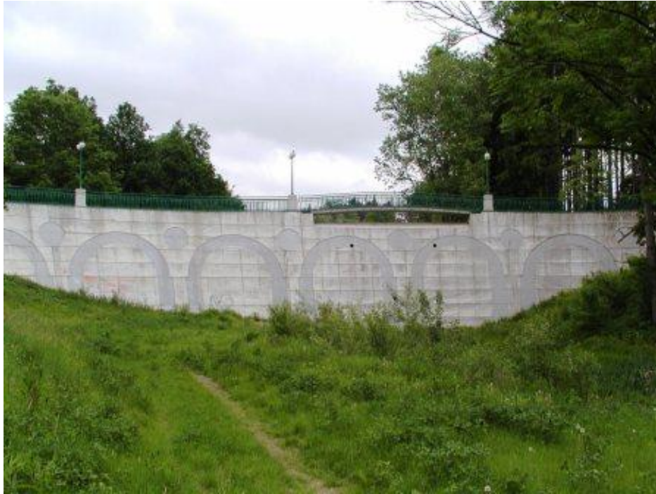
Fig. 2.11 – Hlinky Concrete Gravity dam, height 11m, Czech Republic.
