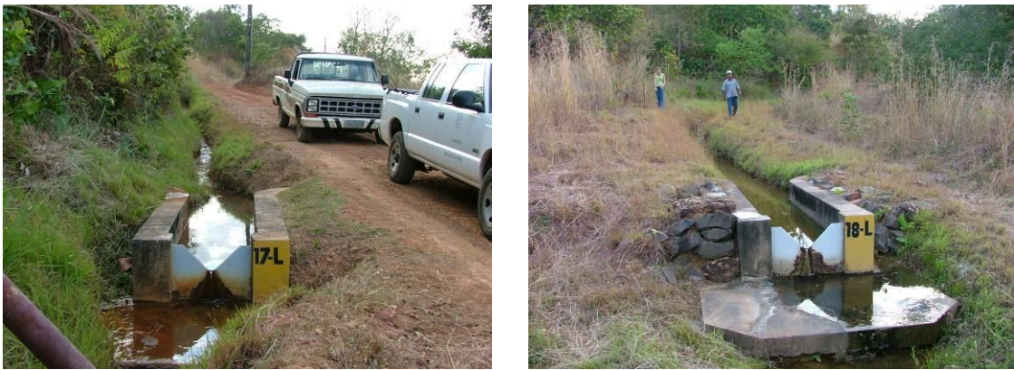
Fig. 6.2 – Leakage measurement using a triangular weir gauge.
