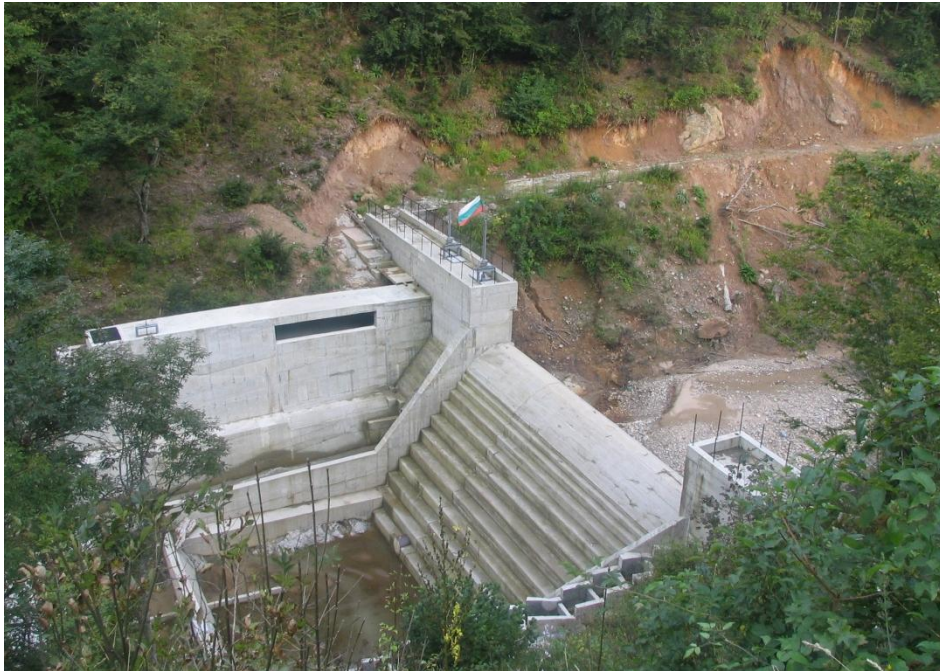
Fig. 2.10 – Lopyan Concrete Gravity dam, 11.60 m height, built in 2004 in Bulgaria
