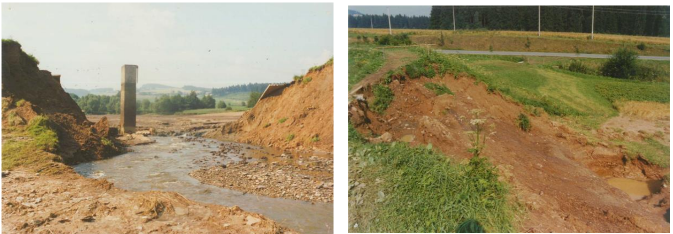
Fig. 4.1 – Busek pond in Czech Republic – dam break after overtopping in August 1991 (extreme summer raining) [2].
