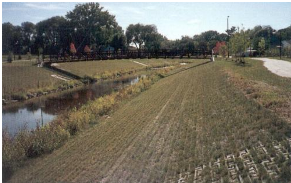
Fig. 7.4 – Lateral slopes protected with concrete blocks and grass
