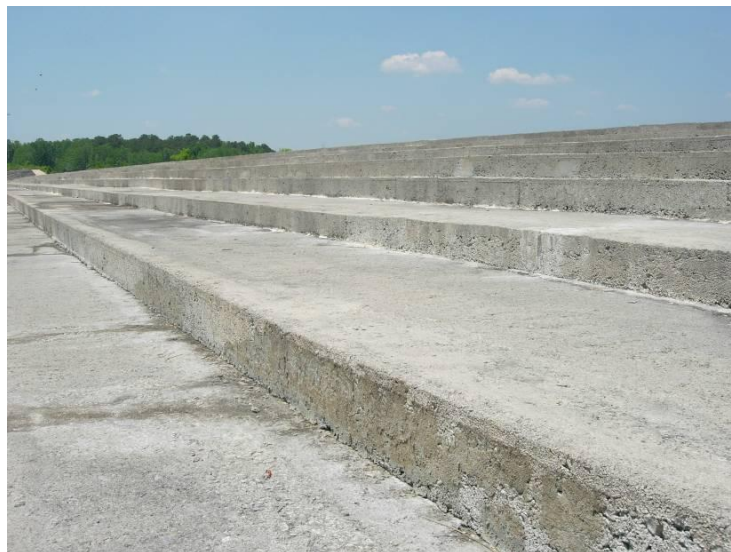
Fig. 7.9 – Excellent condition of RCC steps at Tholocco Lake Dam (Abdo and Adaska/07)
