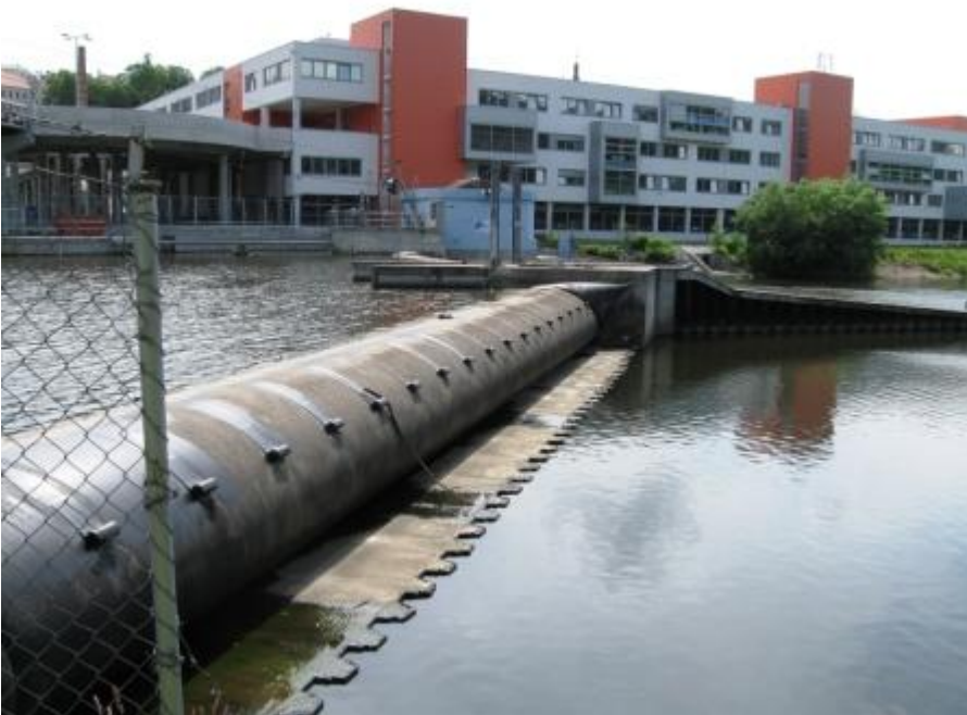
Fig. 18a – Inflatable Small Dam, Mlada Boleslav, Czech Republic
