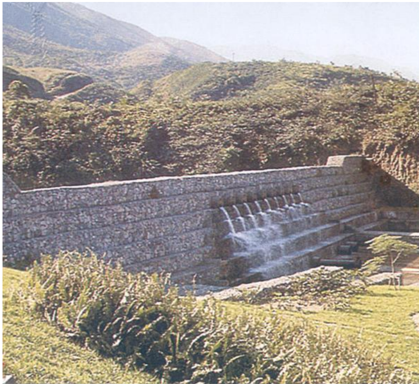
Fig. 2.16 – Gabion dam 12 m high - Brazil
