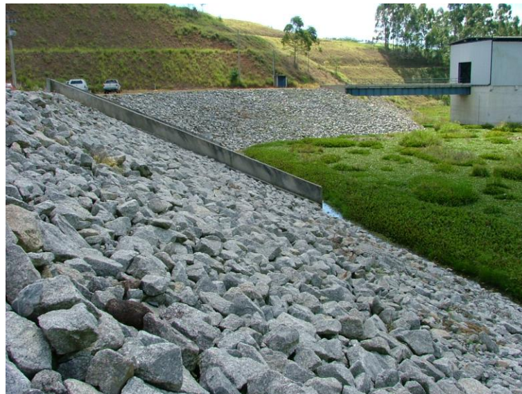
Fig. 5.12 – Upstream gneiss rip-rap at the Paraitinga dam, in Brazil.
