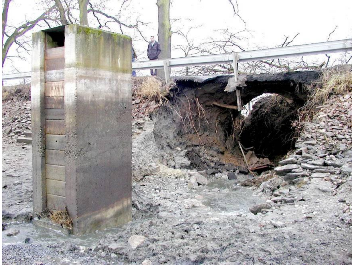
Fig. 3.6 - Cavern in the dam body as a result of wooden bottom outlet decay and internal erosion (Czech Republic)
