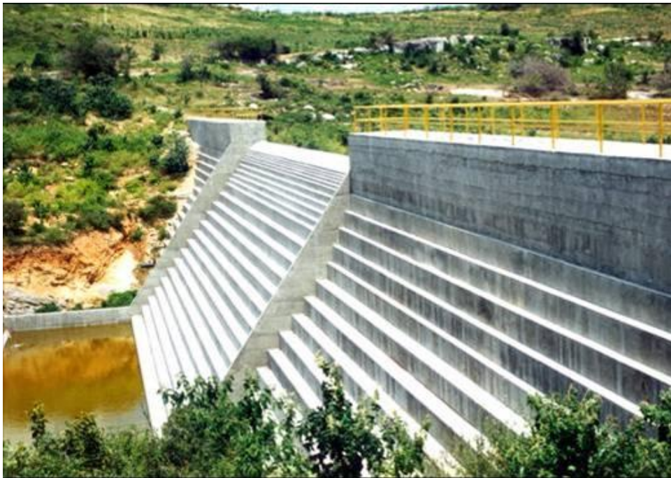
Fig. 2.12 – Trairas RCC concrete dam – Brazil
