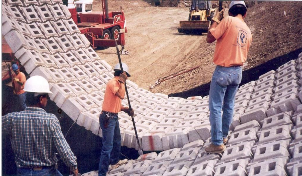
Fig. 7.3 – Installation of the articulated concrete blocks in a channel
