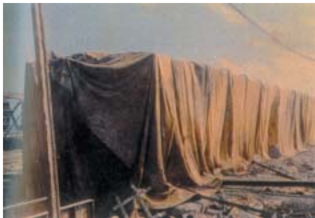
Beam under steam curing.
