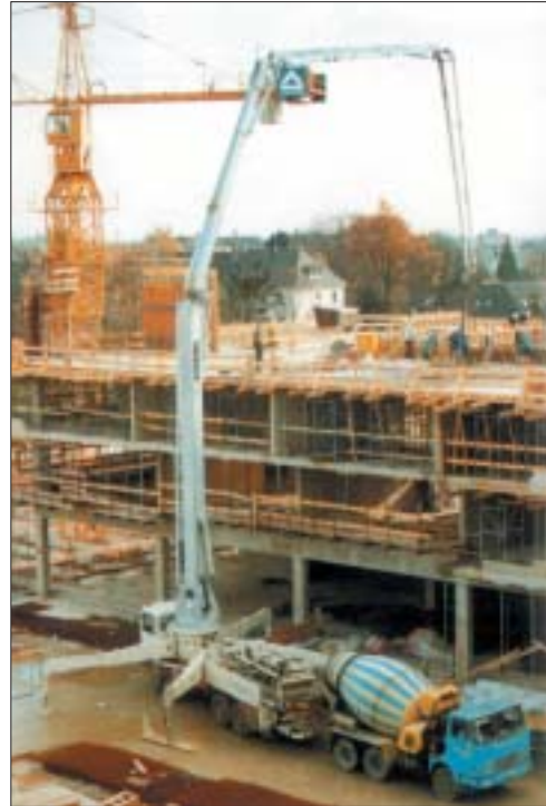
Placing concrete by pump and placing boom.
