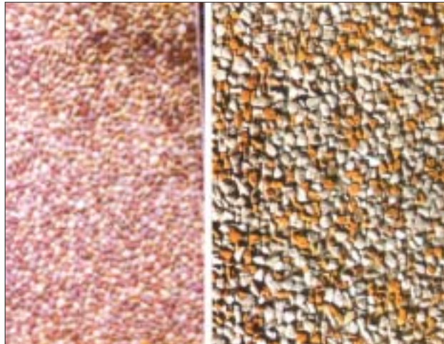
Exposed aggregate finish
