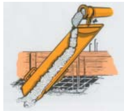
Transporting and placing concrete by chute.
