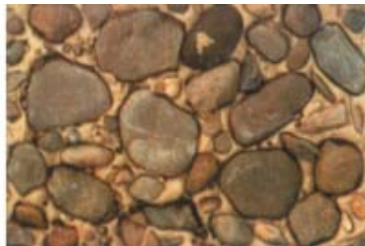
Badly pumpable concrete
