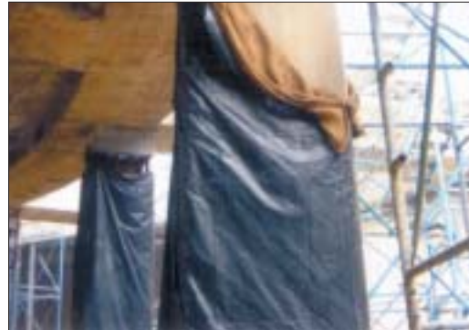
Curing vertical surface by wet covering.
