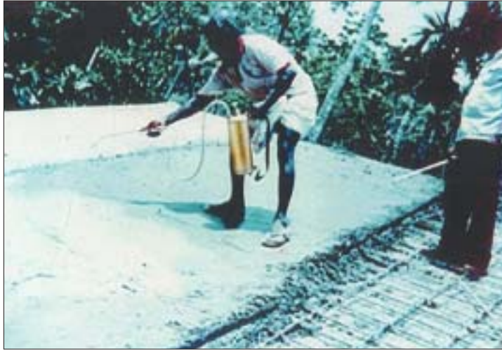
Membrane curing by spraying.
