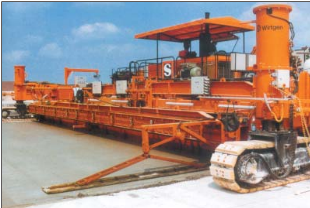
Finishing of road pavement
