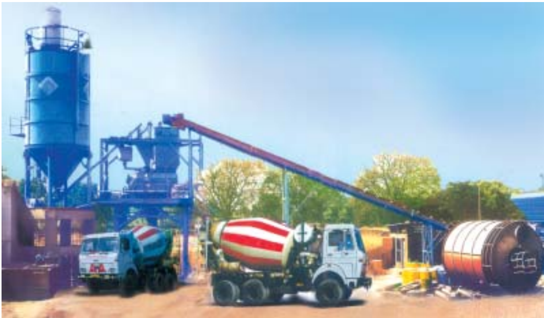
Modern ready mixed concrete plant.
