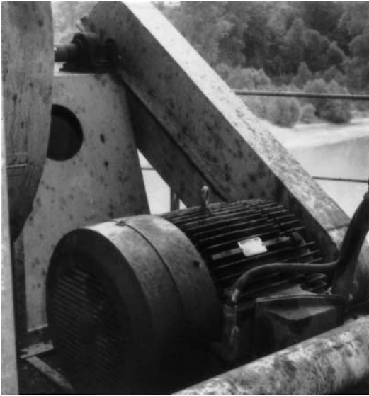
FIG. E-21 Motor-driven barge loading conveyor at a coal handling terminal. (Source: Reliance Electric.)
