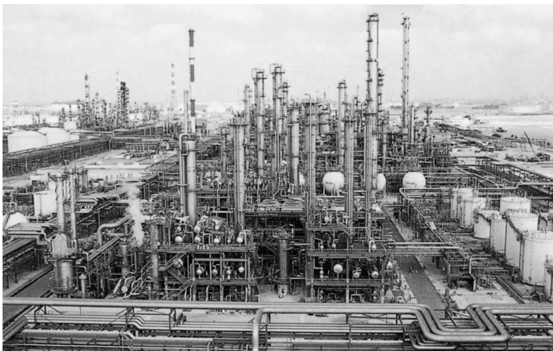
FIG. C-25 PCS II ethylene plant. (Source: Petrochemical Company of Singapore.)
