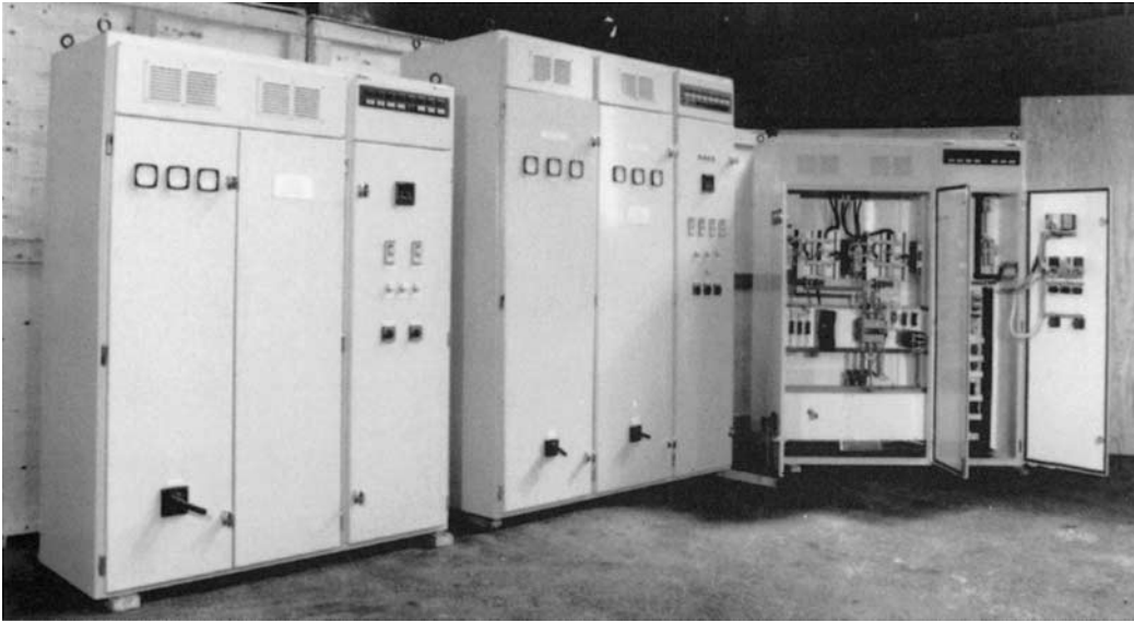
FIG. H-33 Group of three control panels for 200- to 500-kW electric heaters, thyristor controlled. Note separation of control section from power section. (Source: Armstrong Engineering Associates.)
