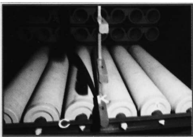
FIG. F-9 Lower tier of filter cartridges is completed. (Source: Peerless.)
