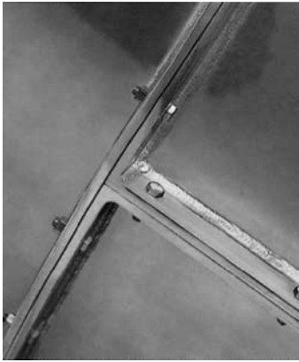
FIG. T-2 Panels are butted together and secured with bolted fasteners on the exterior of the silo. Exterior aluminum structural flanges are \frac{1}{2} in (13 mm) thick and smooth with no ribs or grooves to retain debris. (Source: Peabody TecTank.)
