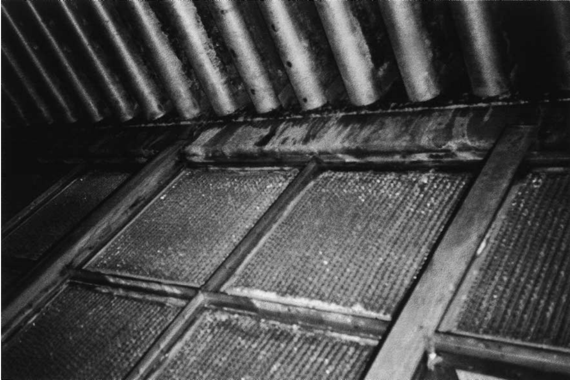
FIG. A-51 Salt penetration through filters. (Source: Altair Filters International Limited.)
