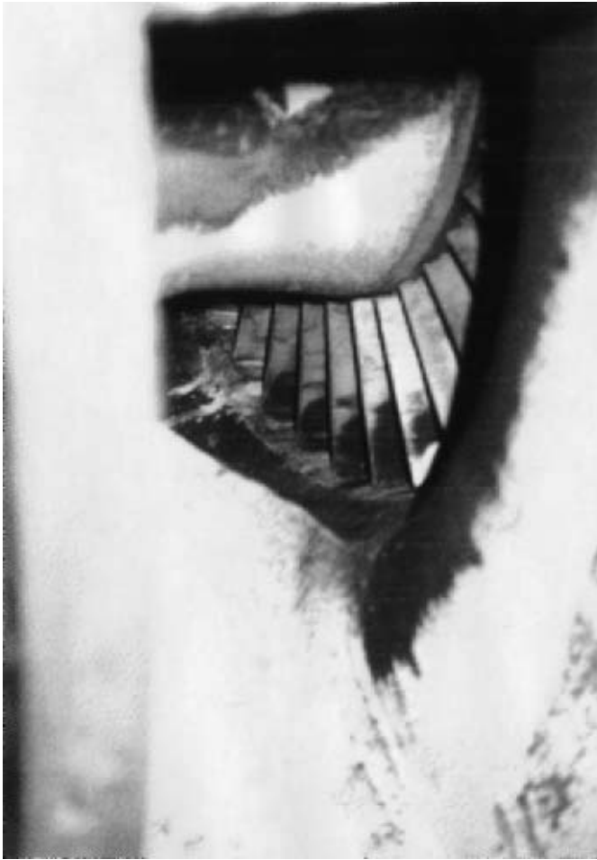
FIG. A-44 Fouling and corrosion. (Source: Altair Filters International Limited.)
