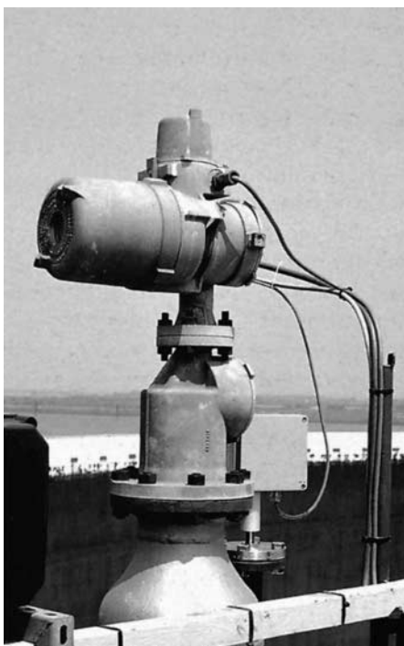
FIG. T-9 Servo gauge. (Source: Enraf.)
