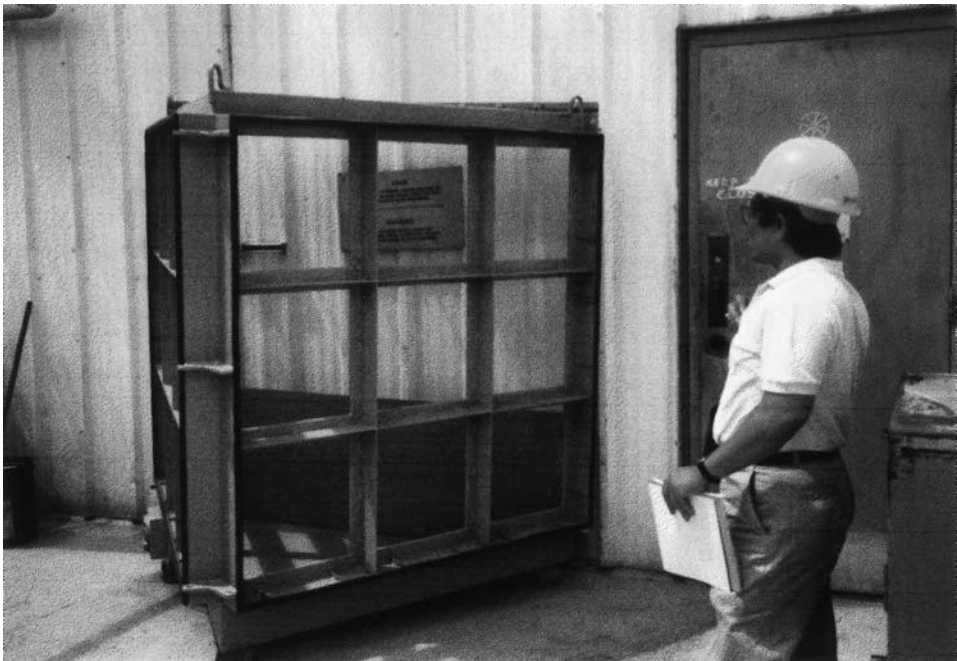
FIG. A-62 A new filter housing awaiting installation. (Source: Altair Filters International Limited.)
