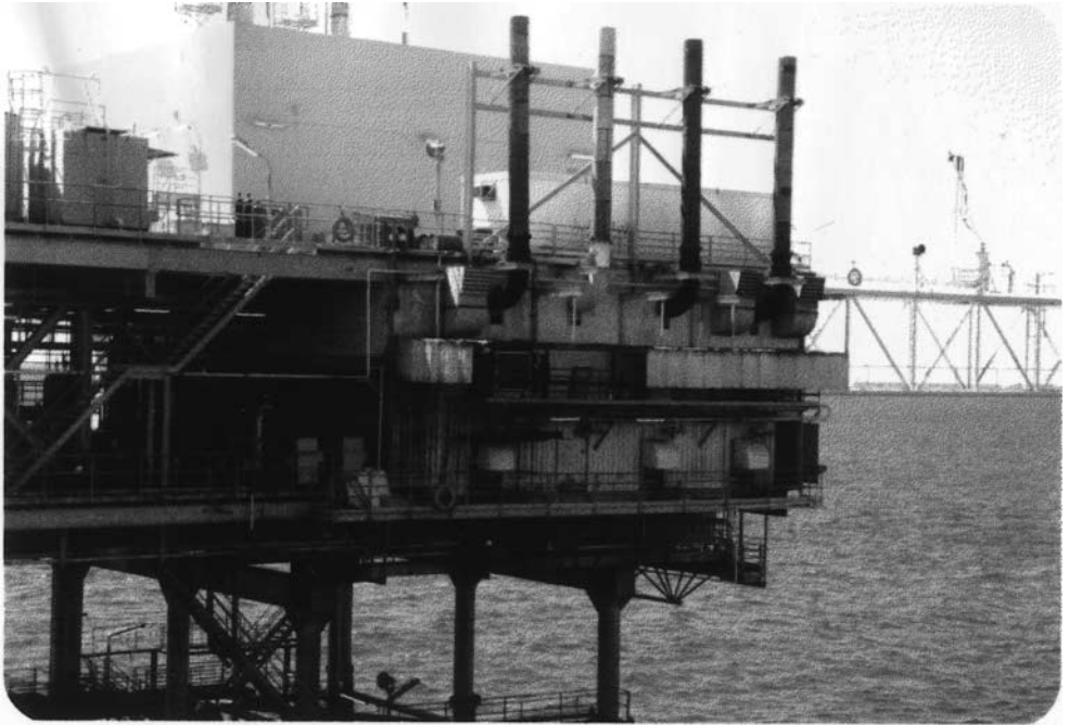
FIG. A-66 Brunei shell petroleum Fairley 4 platform, showing five new filter housings. (Source: Altair Filters International Limited.)
