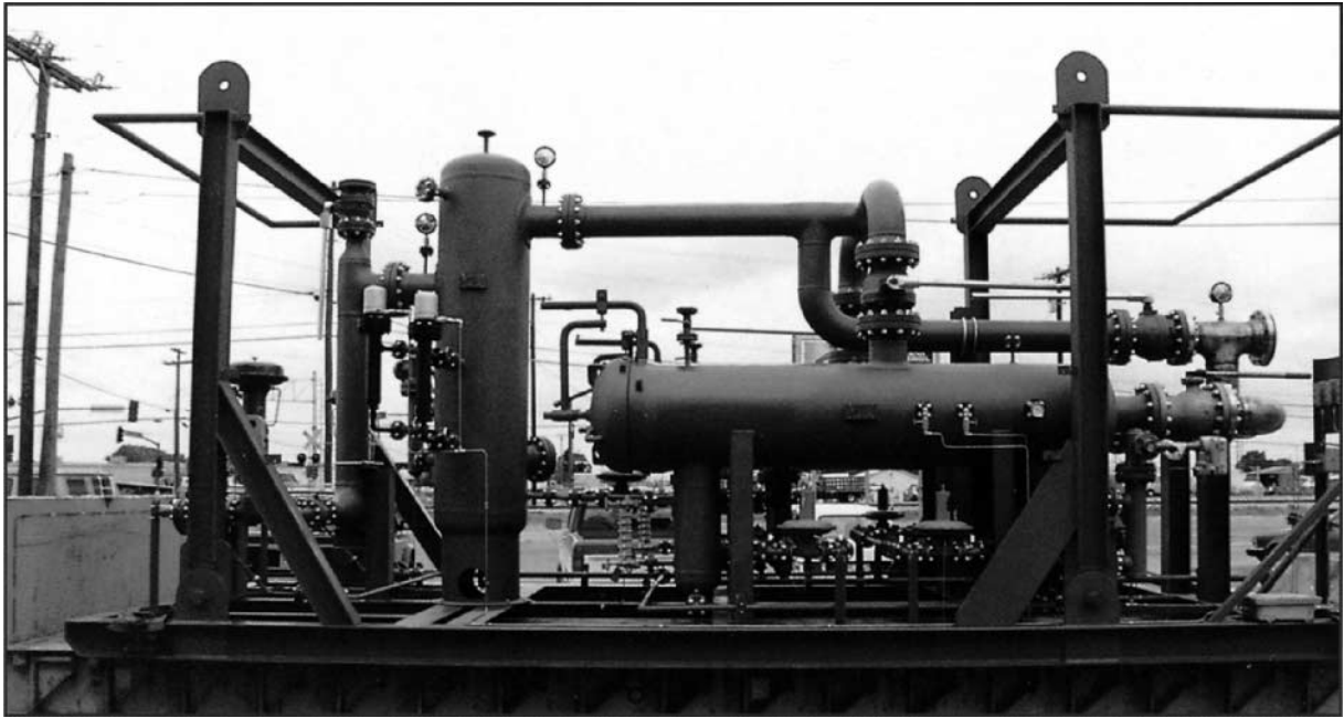
FIG. F-31 A vertical gas separator followed by two duplexed horizontal multitube filters is used to protect two gas turbines in Nigeria. Piping and valves downstream of filters are stainless. (Source: Peerless.)
