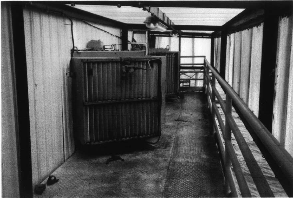
FIG. A-48 Filters protected by a canopy. (Source: Altair Filters International Limited.)
