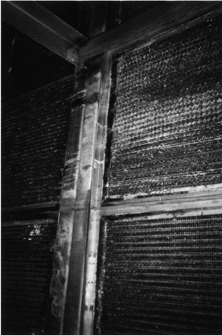
FIG. A-50 Salt penetration through filters. (Source: Altair Filters International Limited.)
