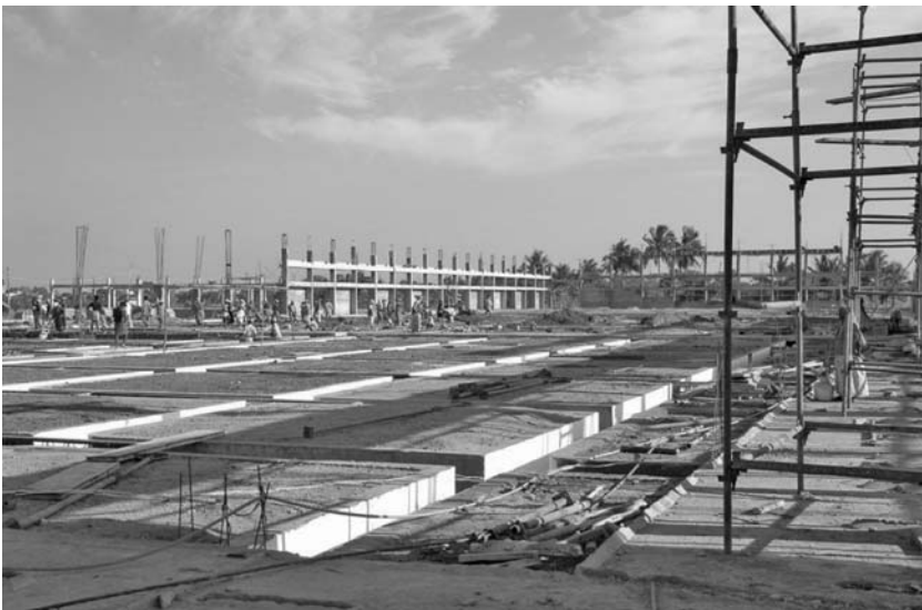
Fig. 10.42 The large floor area within the factory unit
