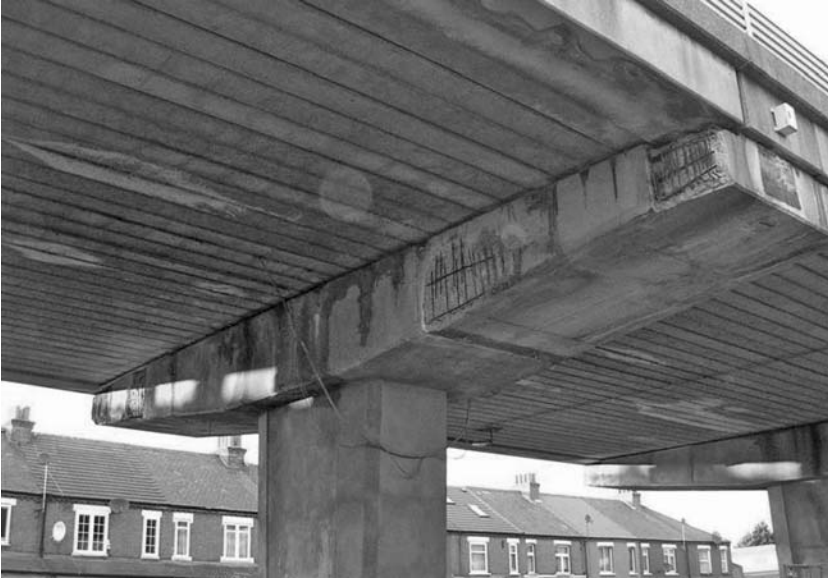
Fig. 10.32 For safety, all loose and delaminated material was removed
