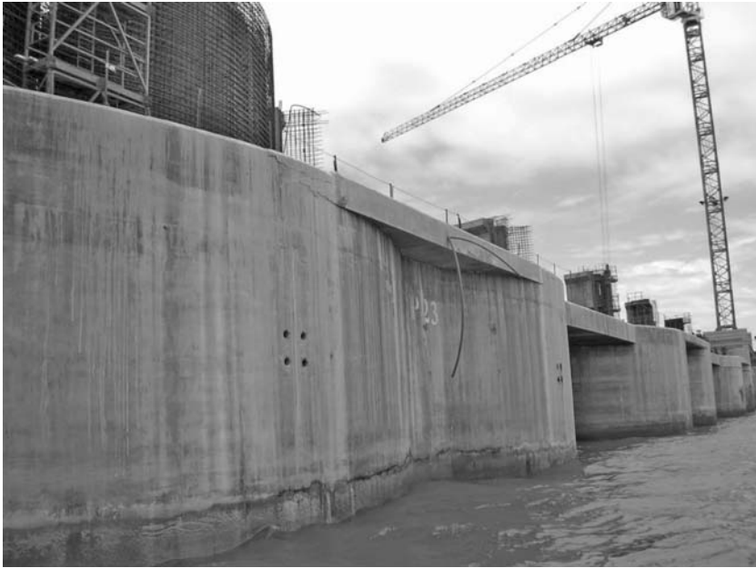
Fig. 10.21 Caissons and the deck slab in place
