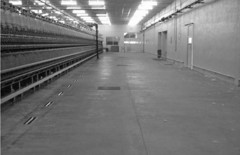
Fig. 10.49 The completed floor in the spinning unit. The polished 'tram tracks' can be seen just in front of the machine. This picture was taken 6 months after production started, and shows no surface wear
