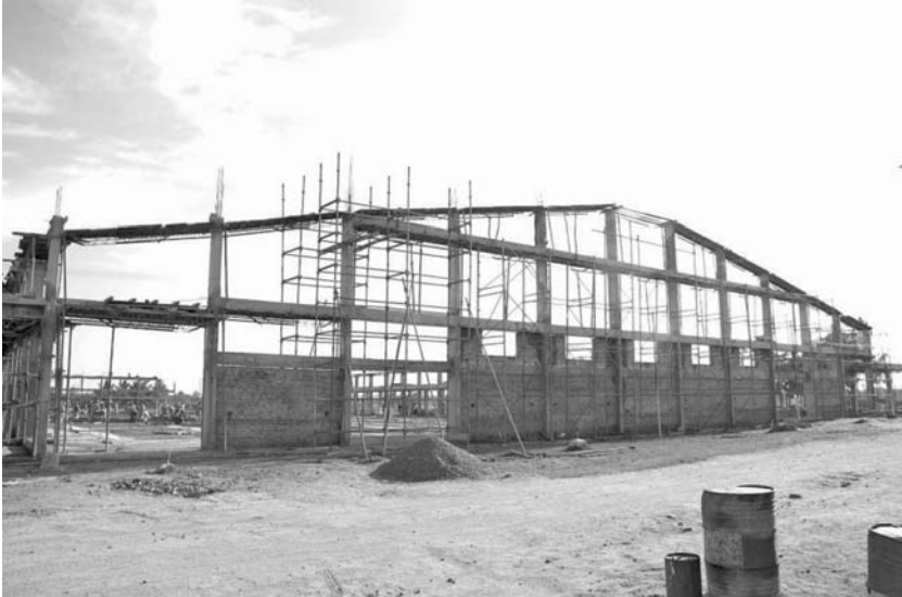
Fig. 10.41 A new factory unit under construction
