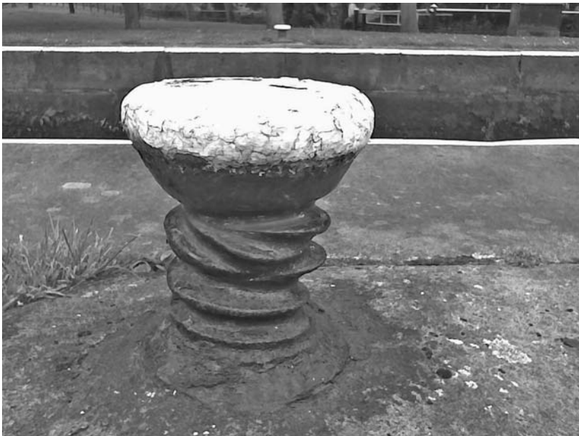
Fig. 3.1 Rope abrading cast iron
