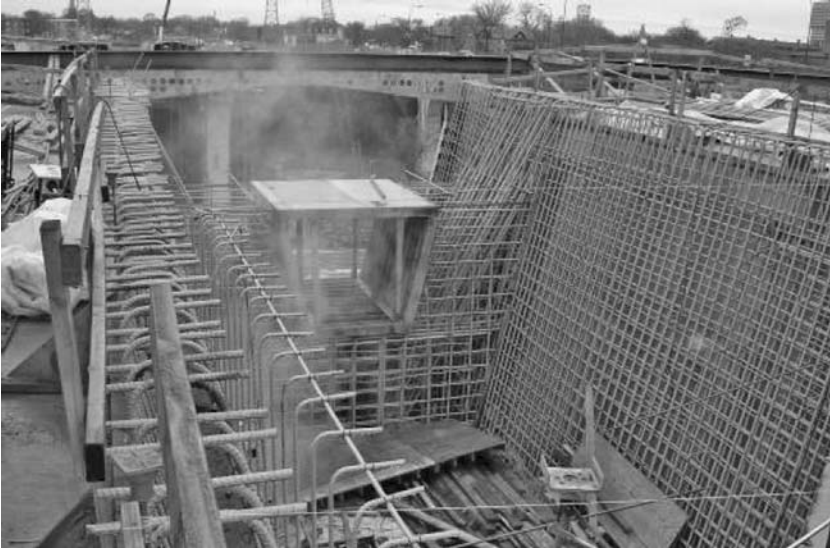
Fig. 7.54 Epoxy-coated reinforcing steel box girder of the I-35 Bridge, Minneapolis
