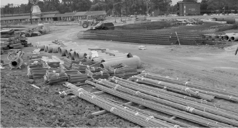
Fig. 7.48 Epoxy-coated reinforcing steel bundled – waiting for placement
