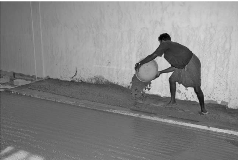
Fig. 10.44 Placing by hand (some larger sites use truckmixers and pumps)
