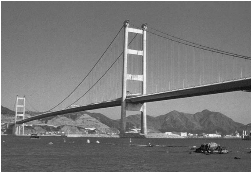
Fig. 10.50 The Tsing Ma Bridge
