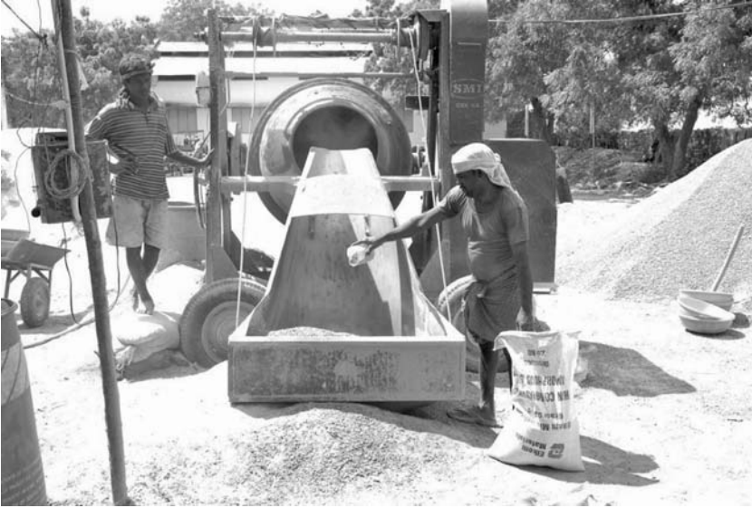
Fig. 10.43 Hand batching into a tumble mixer on site
