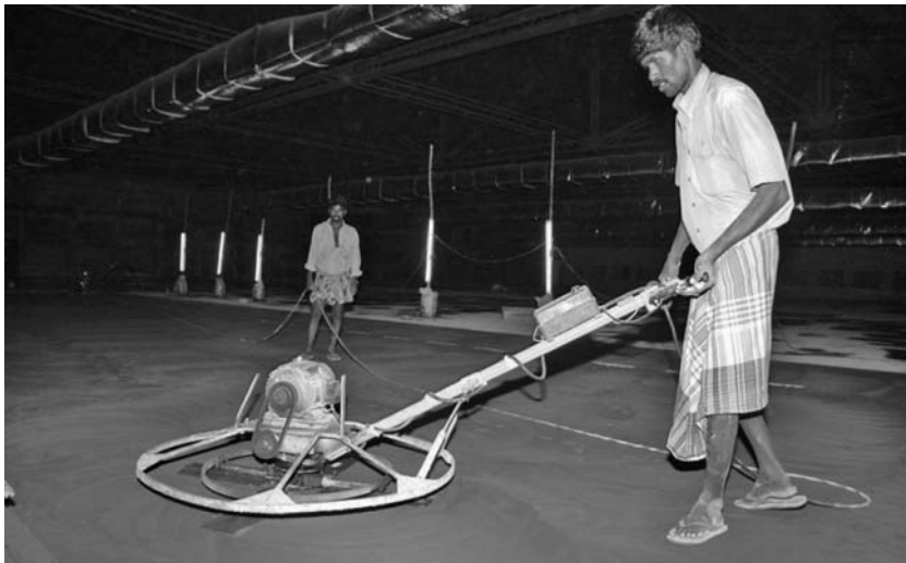
Fig. 10.46 Powerfloating the surface for a solid, sealed finish
