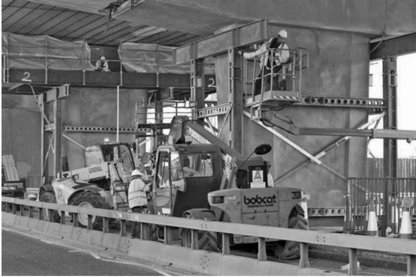
Fig. 10.33 Mesh and overlay cathodic protection can be installed during the day
