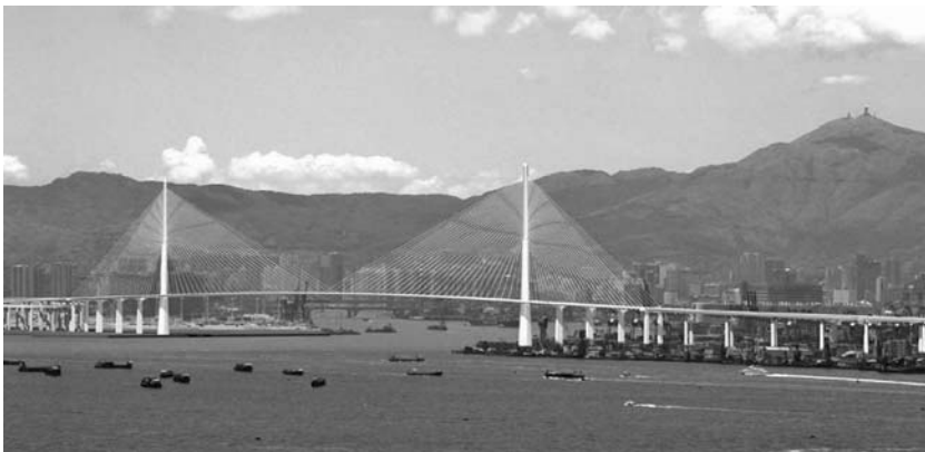
Fig. 9.2 Stonecutters Bridge, Hong Kong, incorporating selective use of stainless steel reinforcement. (Courtesy of Arup)
