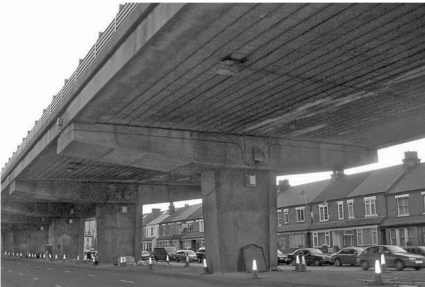
Fig. 10.37 The first four completed installations
