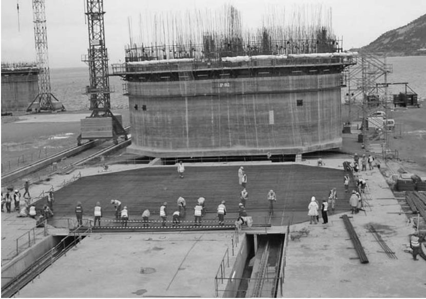
Fig. 10.17 Preparing the casting bed for the base slab of the caisson
