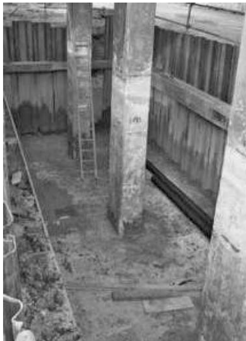
Fig 10.23 Excavation of the slender bridge piers and spread footing
