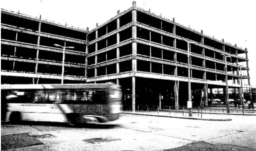
Fig. 1.1 A multi-storey car park in Colchester was pulled down in 1995 because concrete corrosion problems were beyond economic repair
