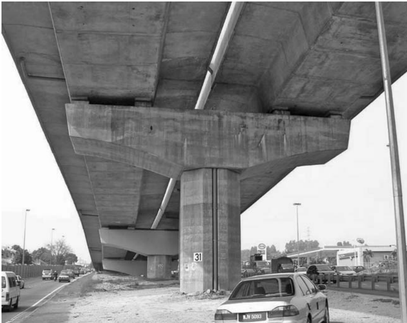
Fig. 10.8 View from beneath the viaduct showing the form on construction
