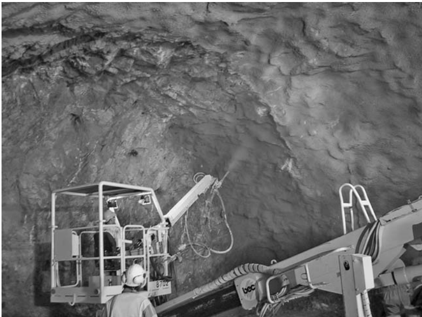
Fig. 7.13 Shotcrete (Fosroc International Ltd)
