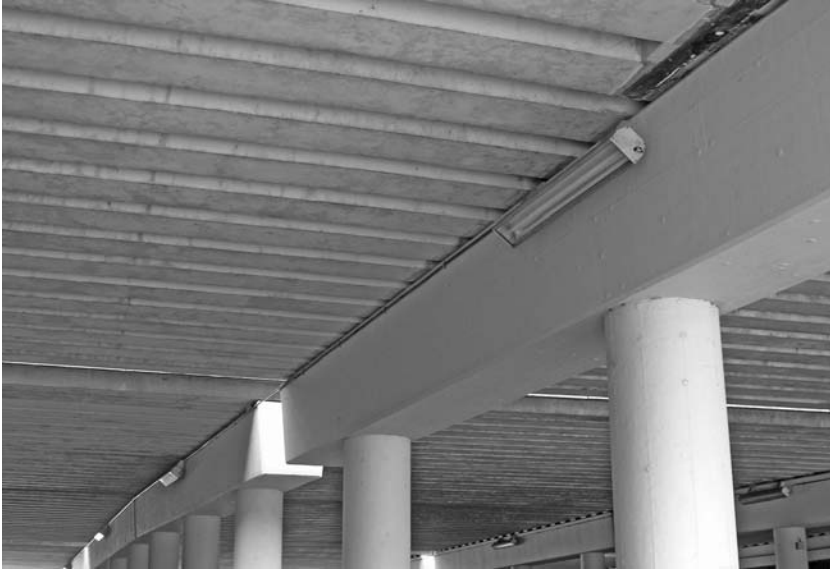
Fig. 11.14 Sheets of zinc hydrogel applied to a bridge substructure. (Reproduced with permission from BAC Corrosion Control Ltd)
