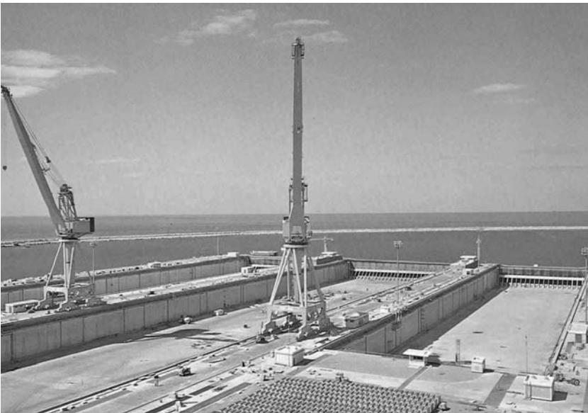
Fig. 10.3 View of the completed dock
