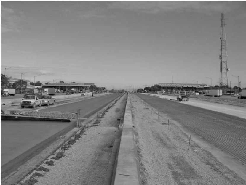
Fig. 7.51 Reconstruction of I-294 western suburbs, Chicago
