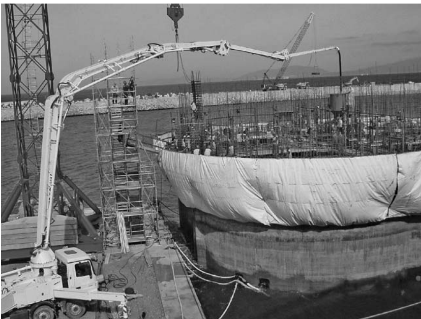
Fig. 10.20 Completing the slipforming at the quayside
