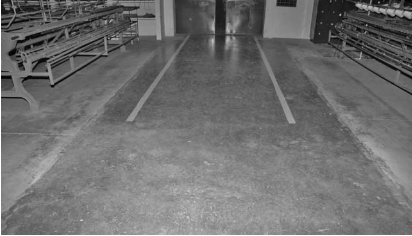
Fig. 10.48 Silica fume concrete refurbishment to worn entranceway
