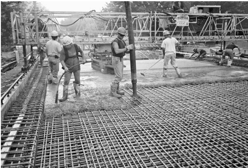
Fig. 7.65 Deck pour – Miles Road Bridge, Cuyahoga County, Ohio
