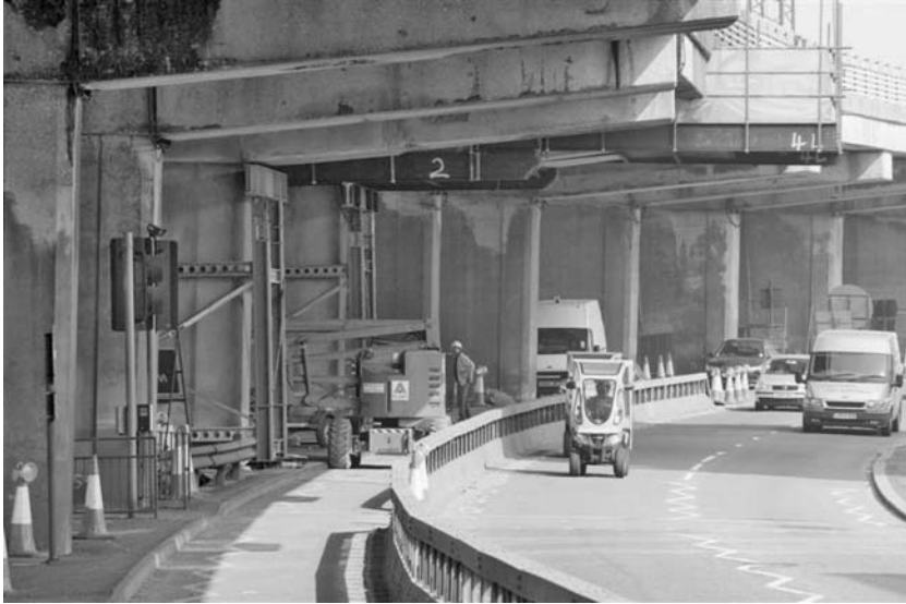
Fig. 10.35 A cantilevered gantry allows coring to proceed over the live carriageway
