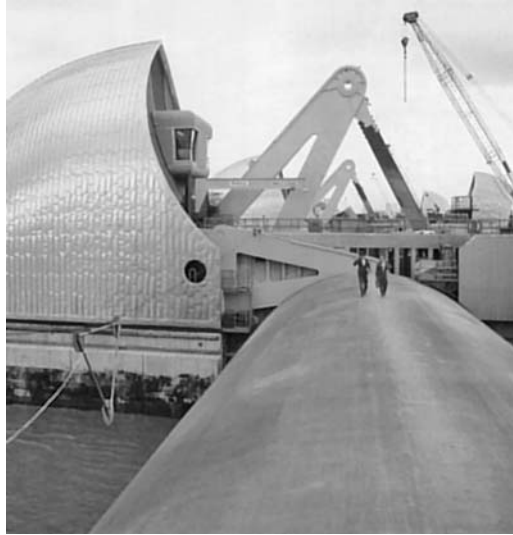
Fig. 7.20 The Thames Barrier
