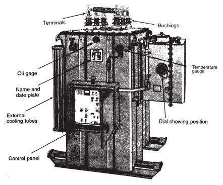
Figure 8-7. A substation voltage regulator.
