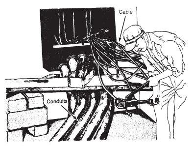
Figure 6-17. A manhole must provide ample headroom for workers.
