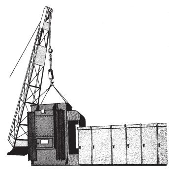
Figure 8-4. A unit substation is conveniently installed.
