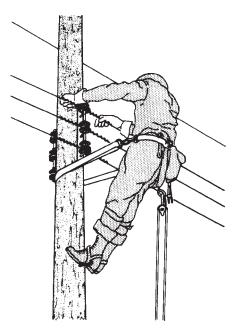
Figure 2-15. A secondary rack holding spool insulators. Lineworker tying wire around insulators on secondary rack.
