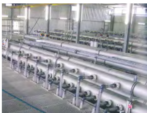
Figure 8.5 membrane installation at the WWTP Nordkanal
