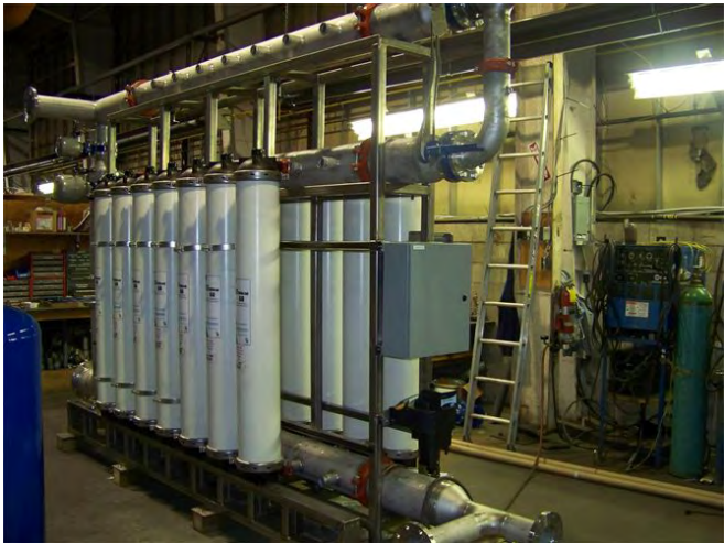
Figure 2.10 MBR. Top: secondary settler; middle: submerged MBR; bottom: cross flow MBR (only membrane module is shown).
