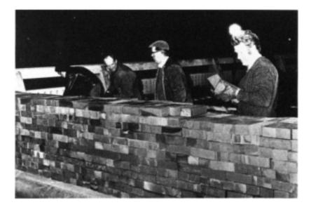
Figure 6.6 Test load on isolated beam using bricks (photograph by courtesy of Professor F.Sawko).
