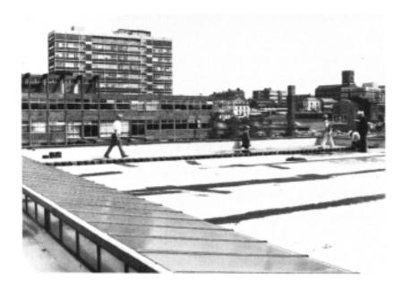
**Figure 6.7** Test load concentrated over roof beam using steel weights (photograph by courtesy of Professor F.Sawko).
