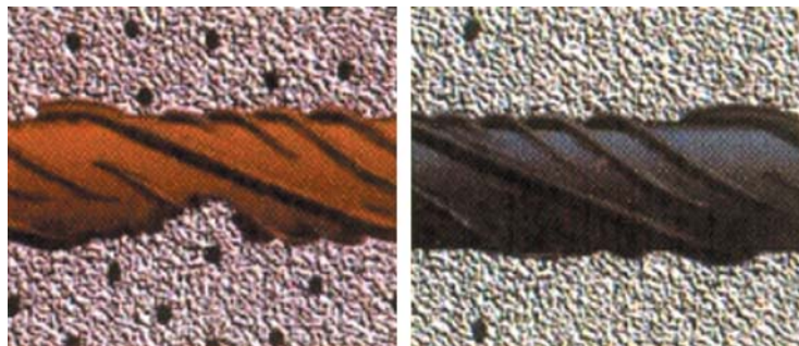
Electro Micrograph showing corrosion in poor concrete
