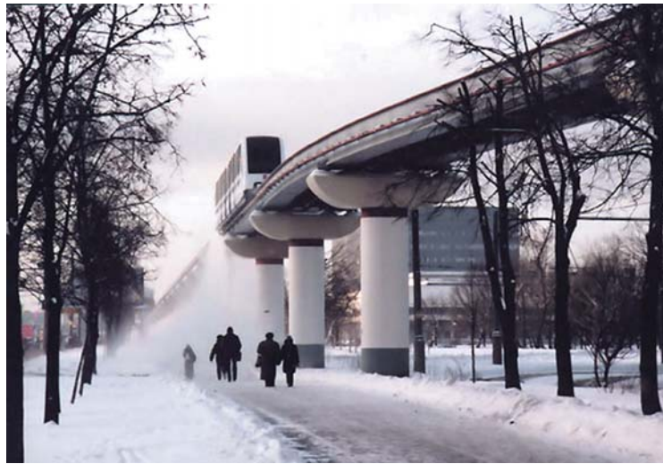
Concrete structures subjected to alternate cycles of freezing and thawing undergoes considerable loss of durability.
