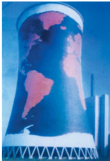
Biggest world map was drawn on cooling tower in Germany using Emce Colour - flex for protection of concrete subjected to aggressive acidic environment.
