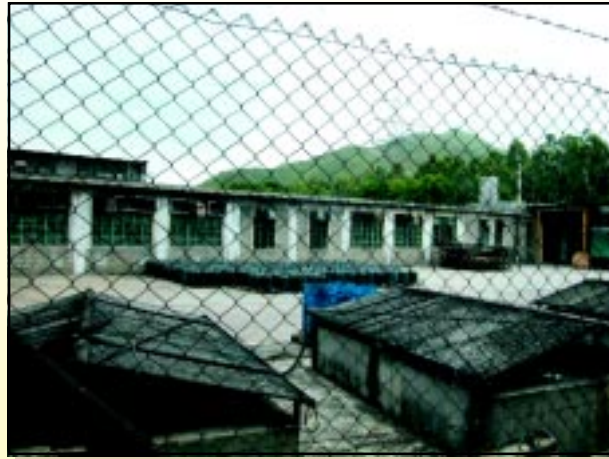
Figure 9 - Fermentation Tanks in the Soya Sauce Factory
