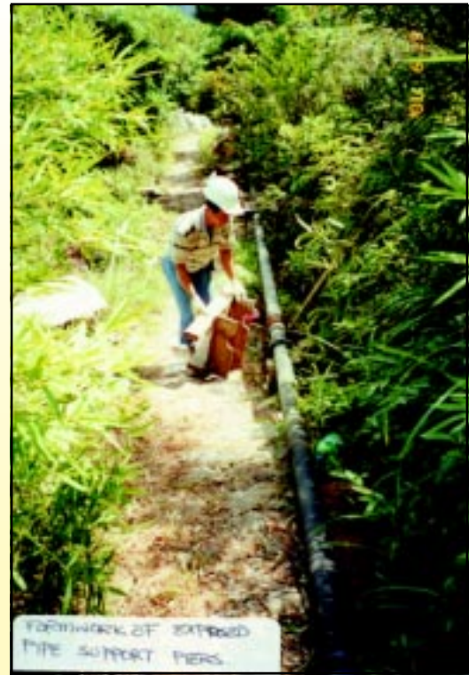
Figure 7 : Exposed D.I. Pipes within Tai Long Wan Archaeological Site
