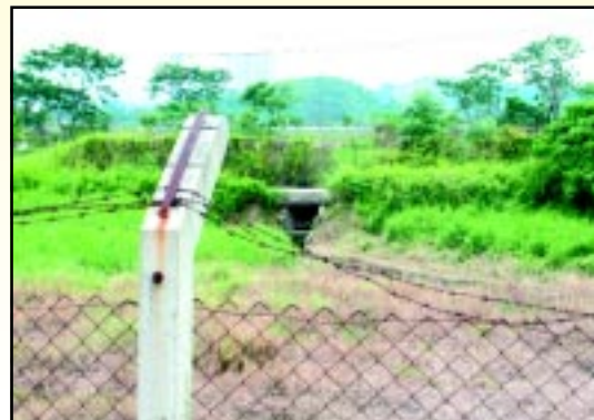
Figure 6 - General View of Existing Vehicular Crossing
