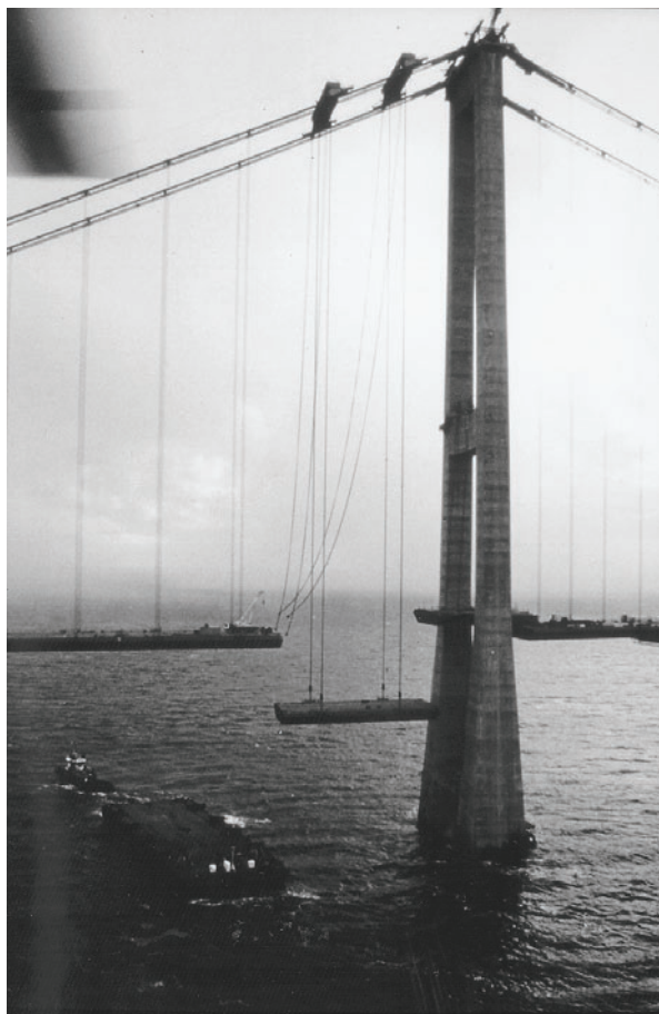
FIGURE 3.13 Great Belt Bridge, Denmark. (Courtesy of Ben C. Gerwick, Inc.)
