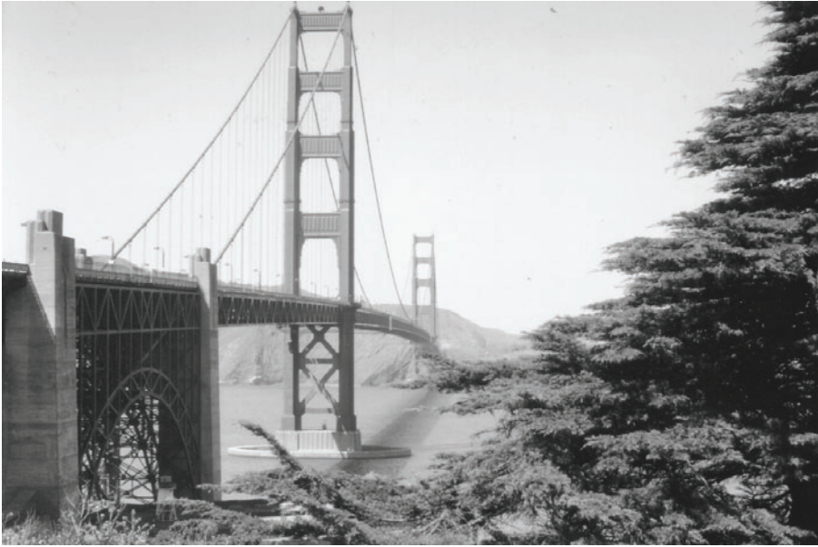
FIGURE 3.1 Golden Gate Bridge, San Francisco. (Courtesy of Charles Seim.)
