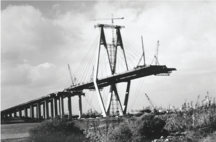
FIGURE 3.10 Baytown Bridge, Texas. (Courtesy of T. Y. Lin International.)
