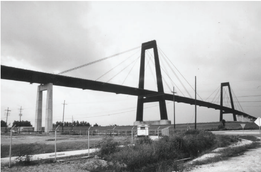
FIGURE 3.6 Luling Bridge, New Orleans, Louisiana. (Courtesy of Charles Seim.)
