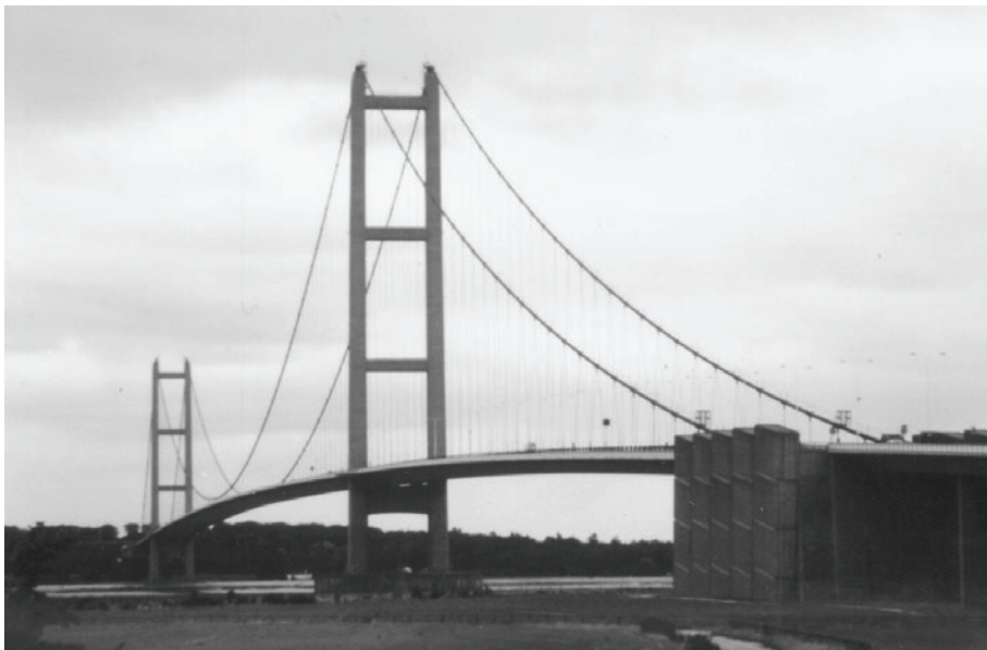
FIGURE 3.12 Humber Bridge, England. (Courtesy of Charles Seim.)
