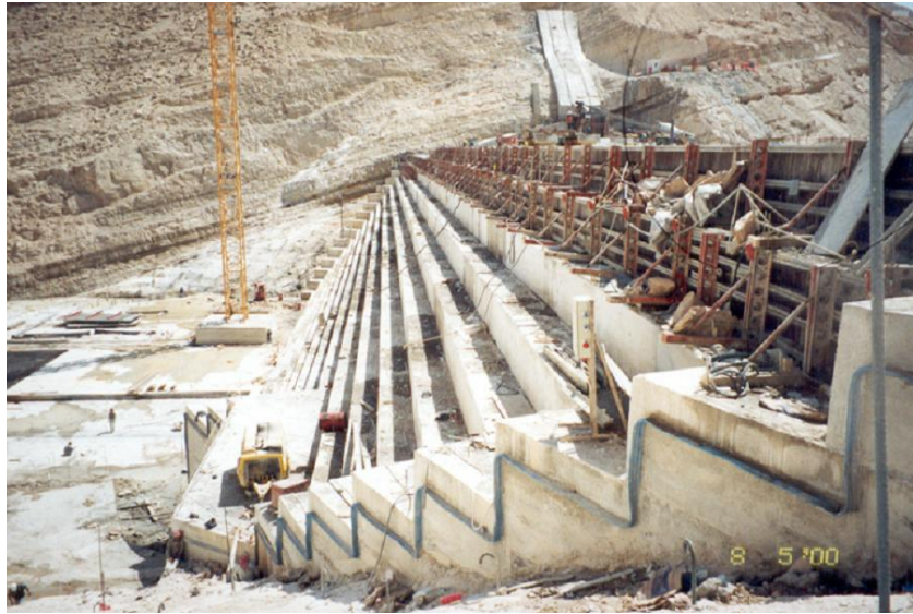
Figure 10. Tannur Dam – Embedded waterstop between GERCC and concrete spillway
