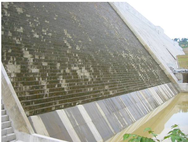
Figure 9. Kinta dam – GERCC faced stepped spillway (about to spill)
