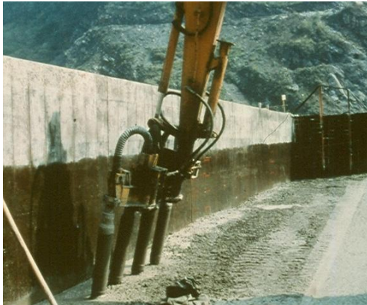
Figure 3. Jiangya dam – Gang mounted vibrators consolidating GERCC
