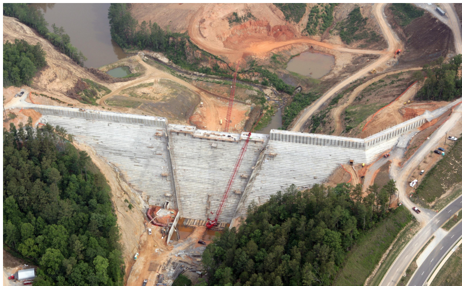
Figure 7. Hickory Log Creek dam – Overview
