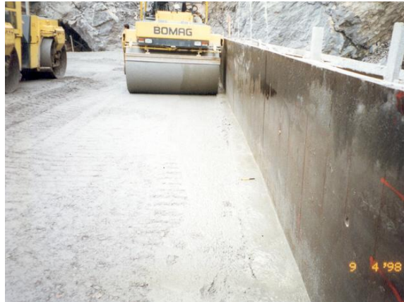
Figure 4. Jiangya dam - Compaction of GERCC / RCC interface
