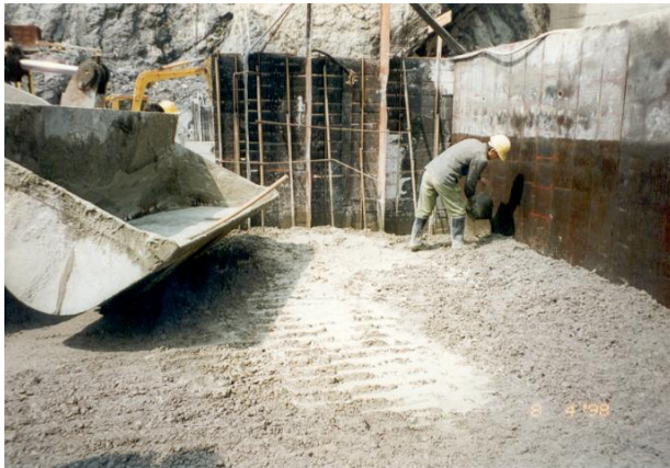
Figure 2. Jiangya dam, laborer applying grout
