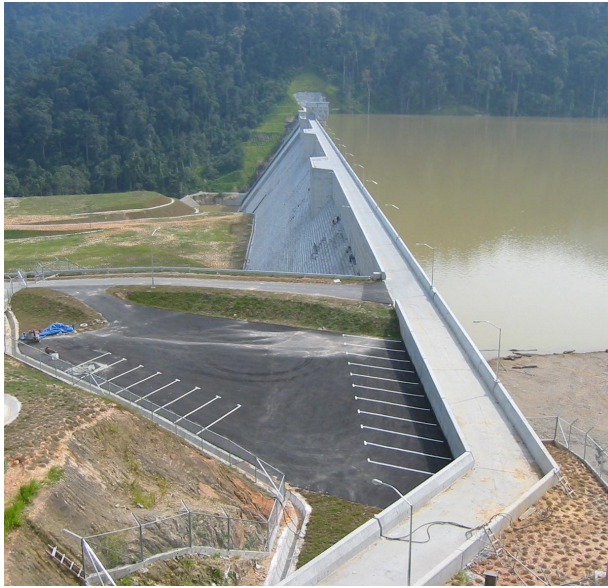
Figure 5. Kinta dam – Overview
