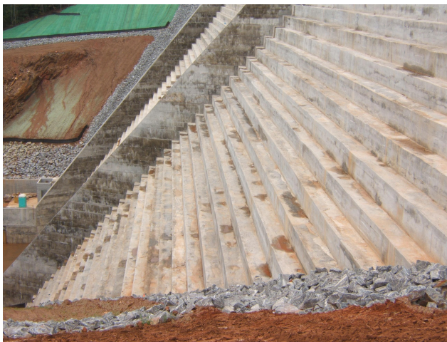
Figure 8 Hickory Log Creek dam – Completed GERCC downstream steps
