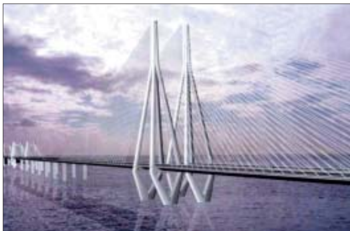
Bandra Worli Sea Link Project - an artist's impression. In this 8 lane bridge 60 MPa concrete is going to be used. Courtesy : Hindustan Construction Company.
