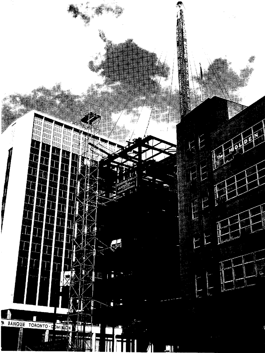
Fig. 33.8 A guy derrick used as a climbing crane
