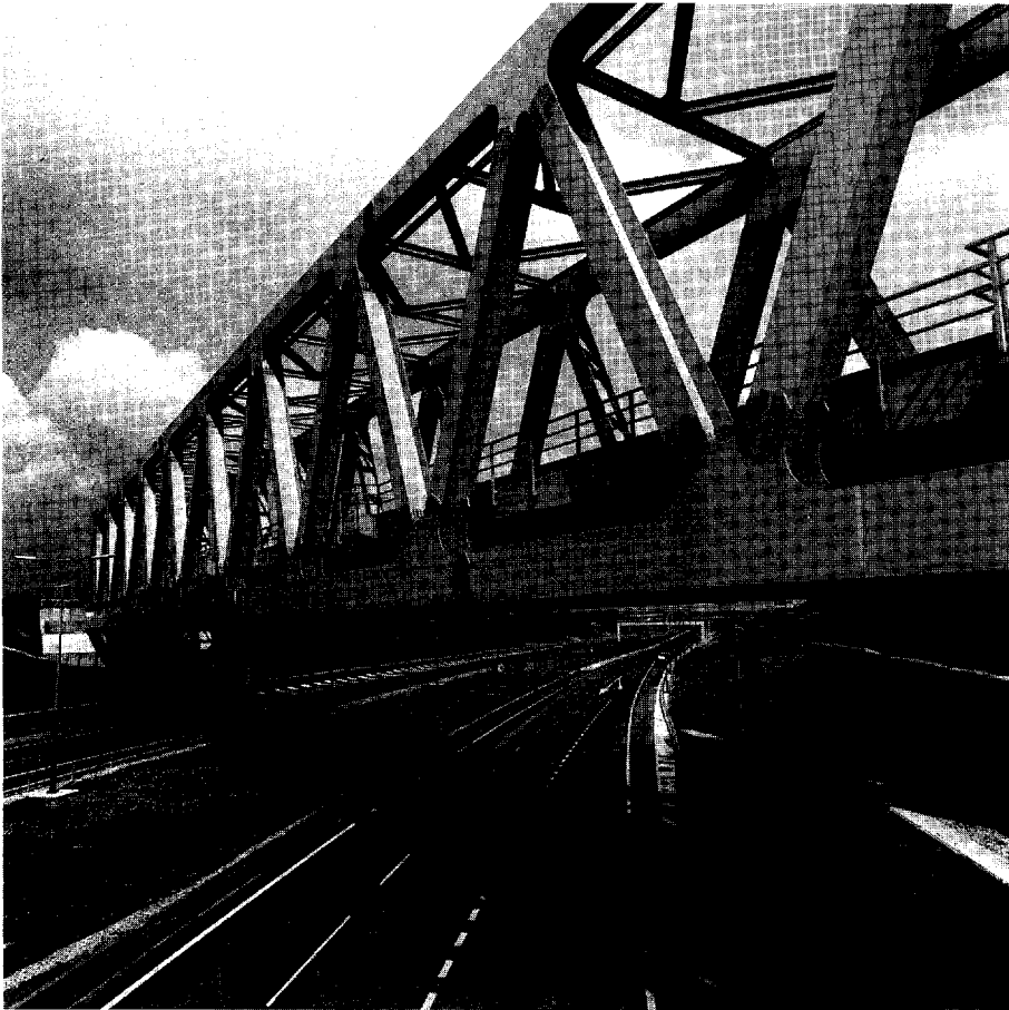
Fig. 19.2 Brinnington Railway Bridge
