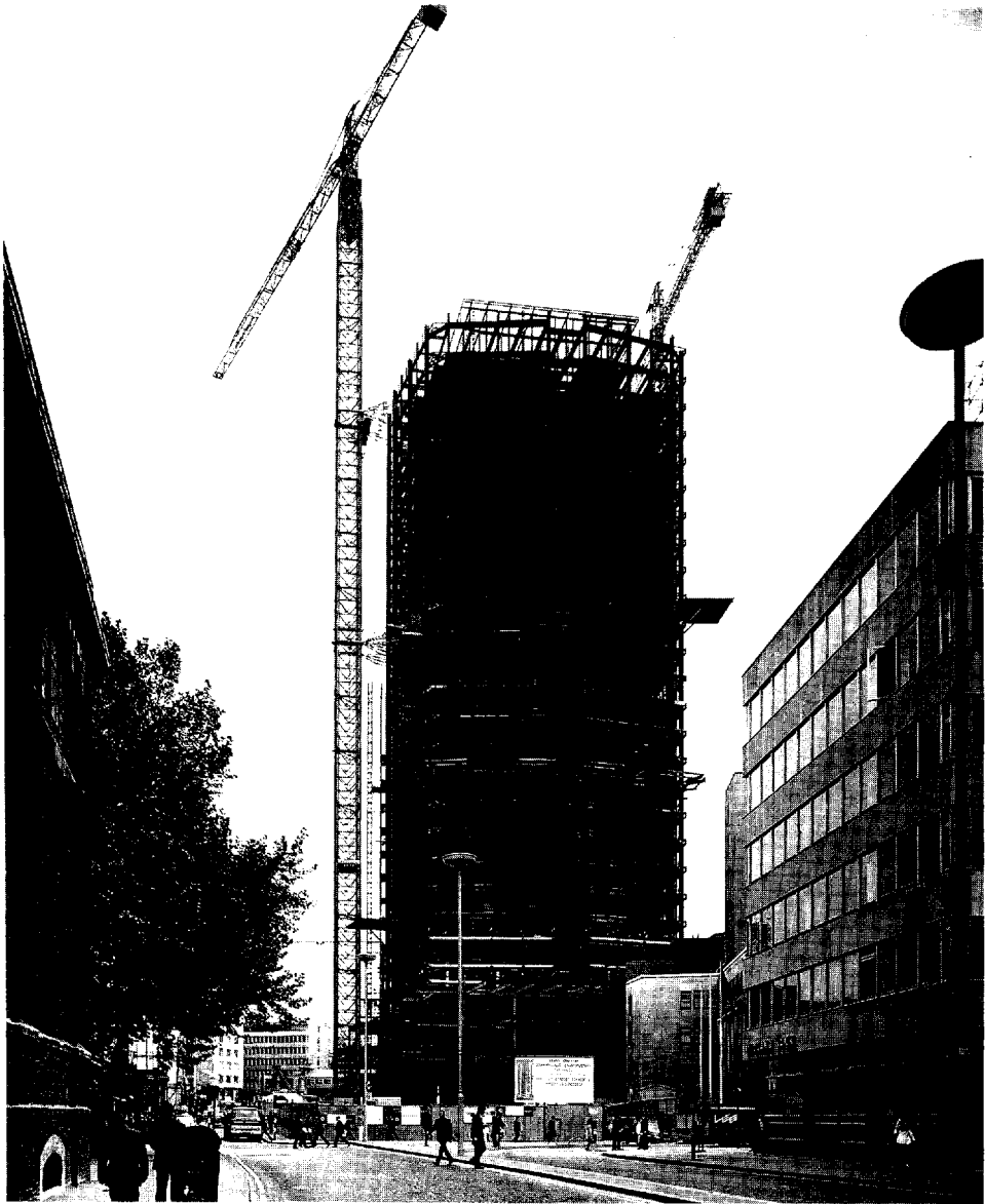
Fig. 33.7 A tower crane tied to the erected structure
