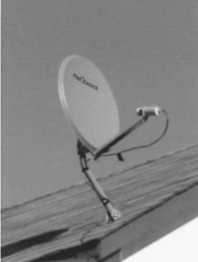
Figure 16.6 A typical DBS antenna installation.
