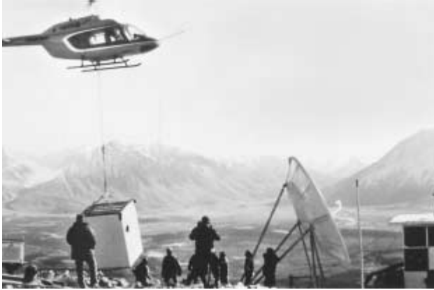
Figure 14.7 Transportable message station. (From Telesat Canada, 1983. )
