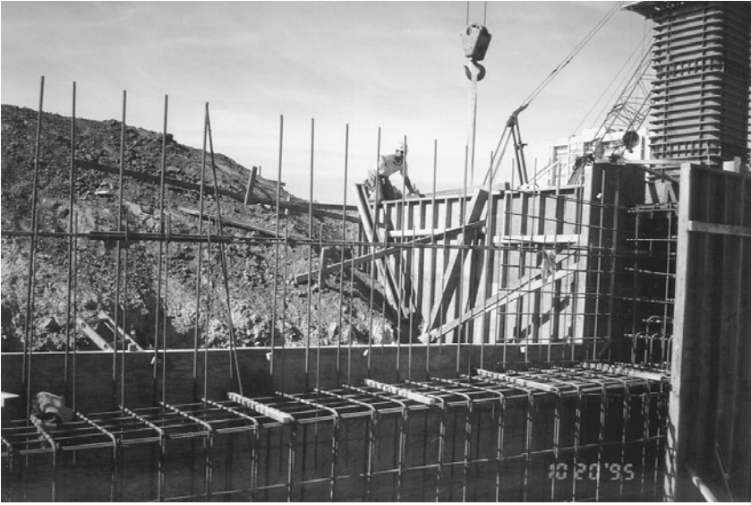
FIGURE 4.3 Wingwall and abutment construction.
