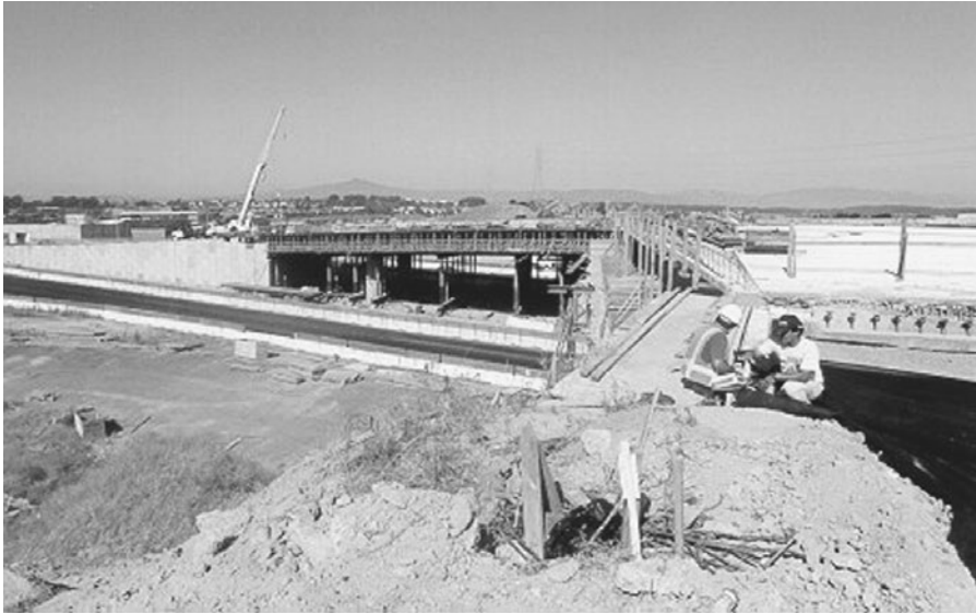
FIGURE 2.6 Falsework at I-80 HOV construction, Richmond, CA.
