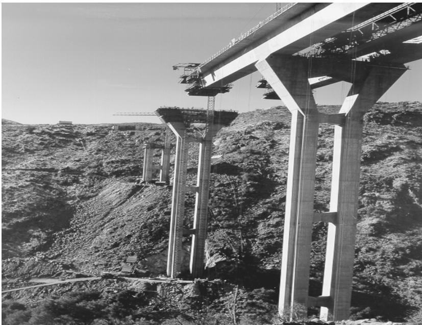
FIGURE 2.3 Pine Valley Creek Bridge — pier construction.
