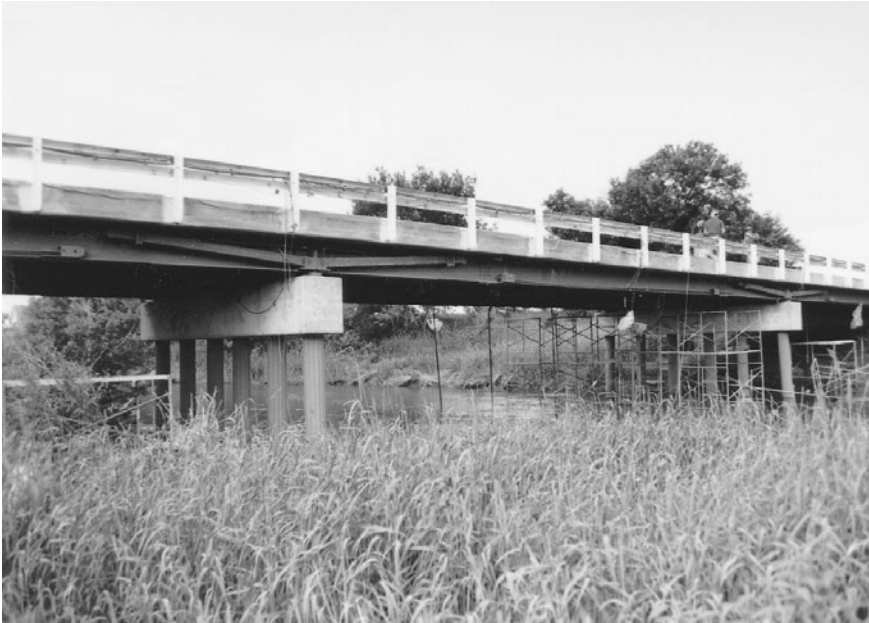
FIGURE 6.26 Photograph of three-span continuous bridge strengthened with post-tensioning and superimposed trusses.
