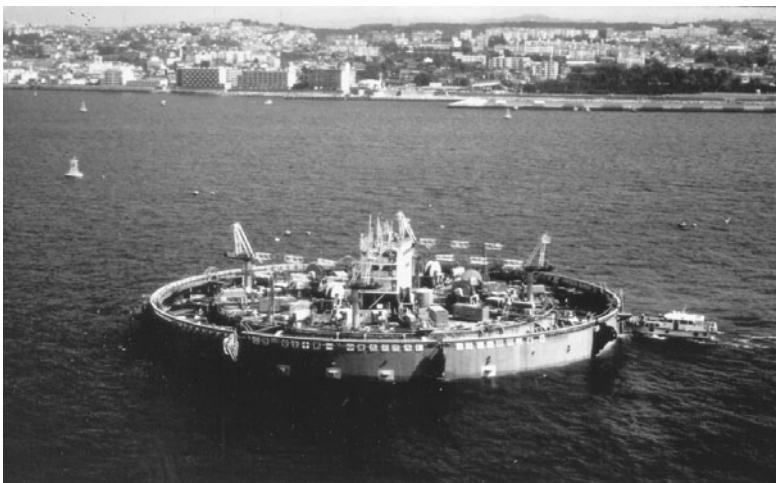
FIGURE 3.20 Akashi Strait Suspension Bridge is founded on steel box caissons filled with tremie concrete.
