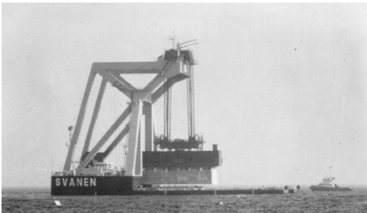
FIGURE 3.31 Setting 7000-ton prefabricated box caisson, Great Belt Western Bridge, Denmark.
