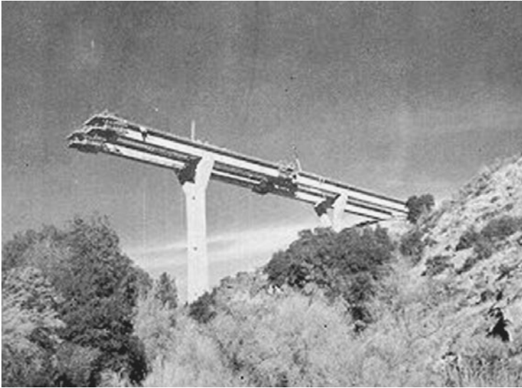
FIGURE 2.2 Pine Valley Creek Bridge — construction at Pier 4.
