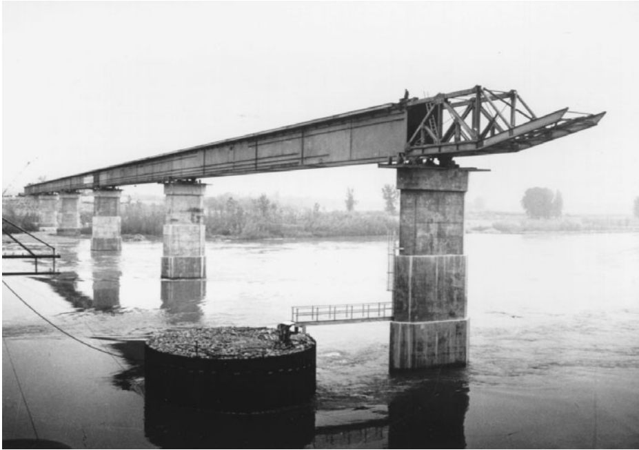
FIGURE 1.41C Leading end of north girder train is now supported on pier 5.
