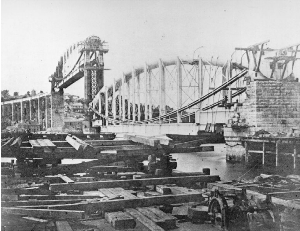
FIGURE 1.14 Royal Albert Bridge across River Tamar, Saltash, England, 1857. The two 455 ft (139 m) main spans, each weighing 1060 tons, were constructed on shore, floated out on pairs of barges, and hoisted about 100 ft (30 m) to their final position using hydraulic jacks. Pier masonry was built up after each 3 ft (1 m) lift.
