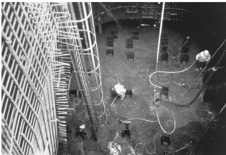
FIGURE 3.13 Pumped-out cofferdam showing tremie concrete seal and predriven steel H-piles.
