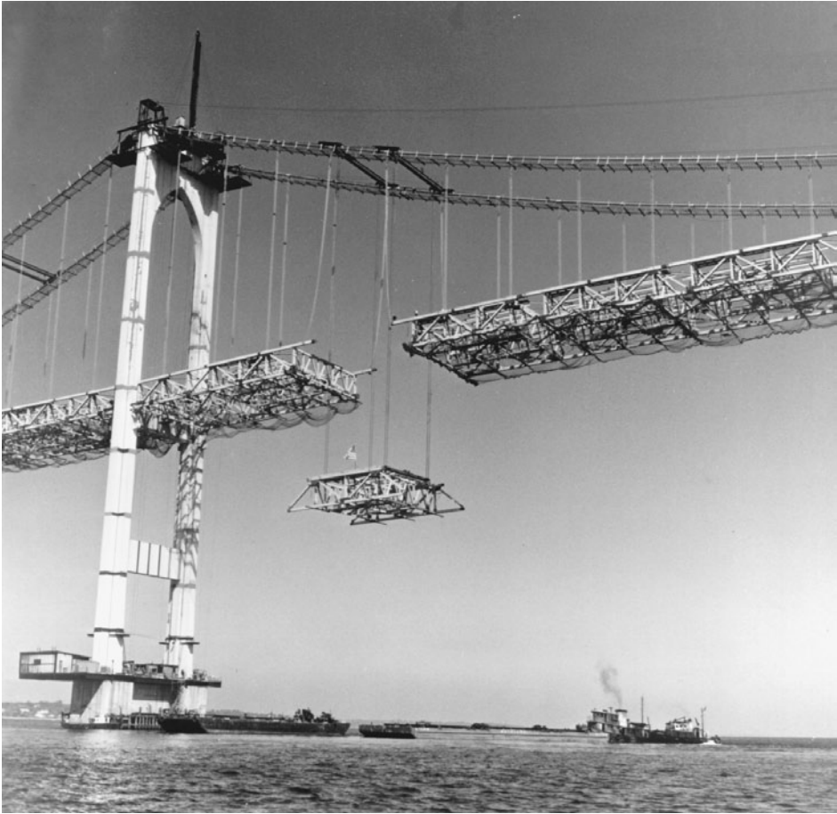
FIGURE 1.40 Suspended deck steelwork erection, Newport Bridge suspension spans, Narragansett Bay, R.I., 1968. Closing mainspan deck section is being raised into position by two cable travelers, each made up of a pair of 36 in. (0.91 m) wide-flange rolled beams that ride cables on wooden wheels. Closing section is 40-1/2 ft (12 m) long at top-chord level, 66 ft (20 m) wide and 16 ft (5 m) deep, and weighs about 140 tons. (Courtesy of Bethlehem Steel Corporation.)
