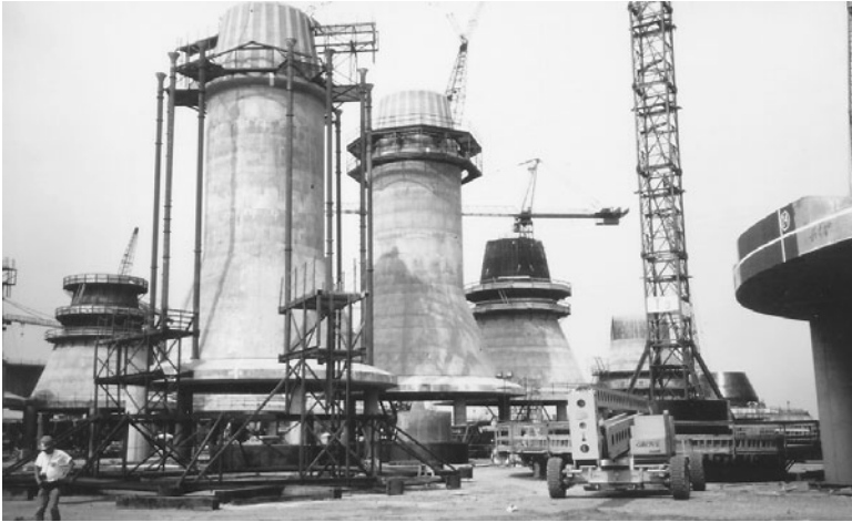
FIGURE 3.25 Prefabrication of pier bases, Prince Edward Island Bridge, Canada.
