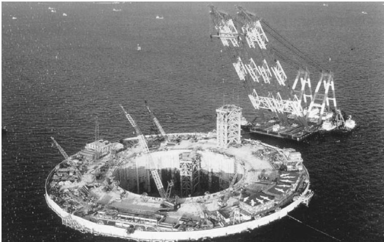
FIGURE 3.10 Slurry wall cofferdam for Kawasaki Island ventilation shaft, Trans-Tokyo Bay tunnels and bridge.
