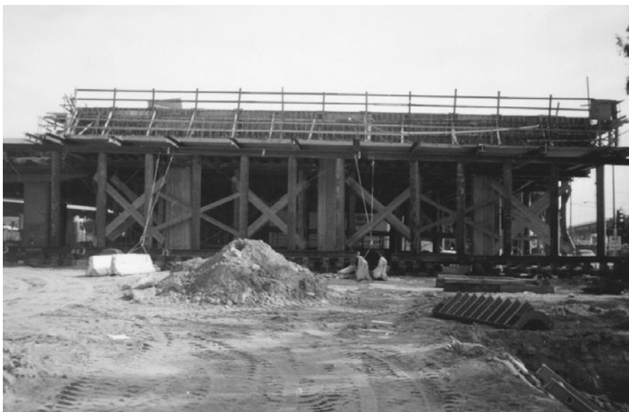
FIGURE 4.10 FW system for cast-in-place concrete bridge.
