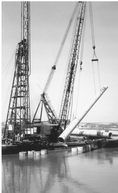
FIGURE 3.6 Large-diameter prestressed concrete pile, Napa River Bridge, California.
