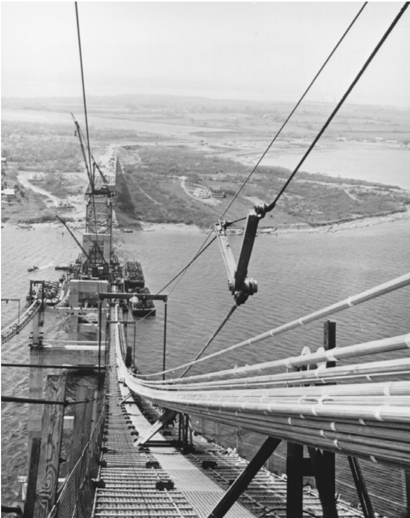
FIGURE 1.37A Aerial tramway tows PWS from west anchorage up side span, then on across other spans to east anchorage. Strands are about 1-3/4 in. (44 mm) in diameter.
