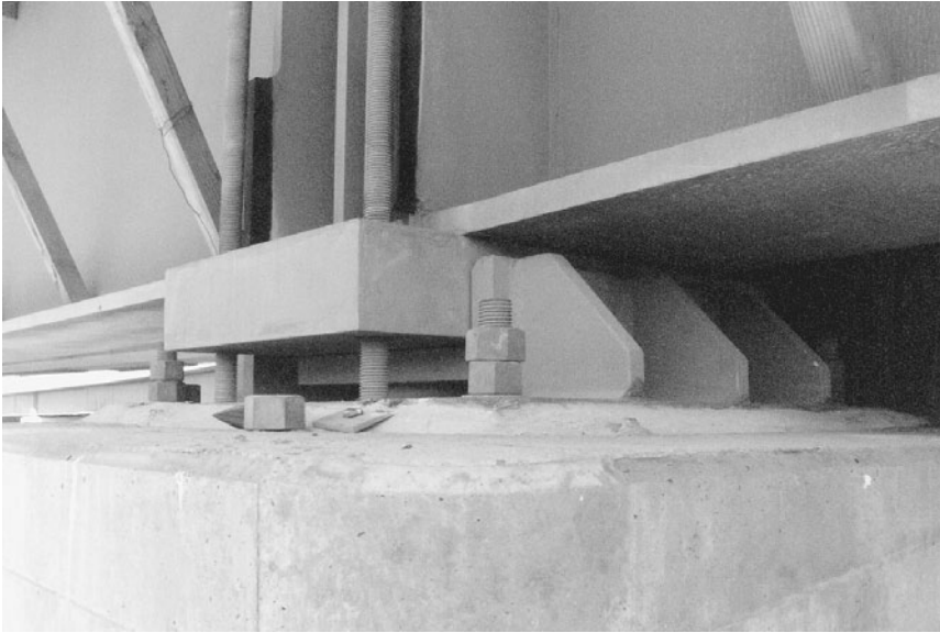
FIGURE 4.8 Bearing assembly of steel plate girder.
