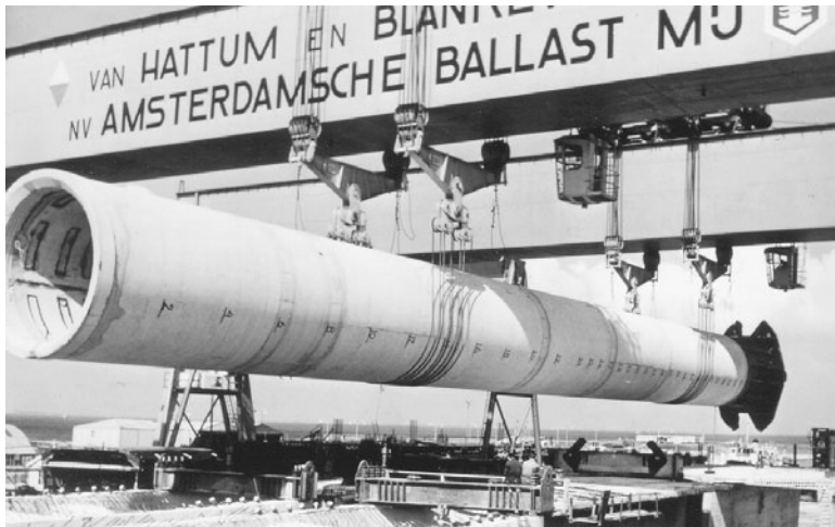
FIGURE 3.7 Prestressed concrete cylinder pile for Oosterschelde Bridge, the Netherlands.
