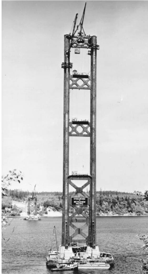
FIGURE 1.24 Tower erection, second Tacoma Narrows Bridge, Washington, 1949. This bridge replaced first Tacoma Narrows bridge, which blew down in a 40 mph (18 m/sec) wind in 1940. Tower legs are 60 ft (18 m) on centers and 462 ft (141 m) high. Creeper traveler is shown erecting west tower, in background. On east tower, creeper erected a Chicago boom at top of south leg; this boom dismantled creeper, then erected tower-top bracing and a stiffleg derrick, which proceeded to dismantle Chicago boom. Tower manhoist can be seen at second-from-topmost landing platform. Riveting cages are approaching top of tower. Note tower-base erection kneebraces, required to ensure tower stability in free-standing condition (see Figure 1.27 ).
