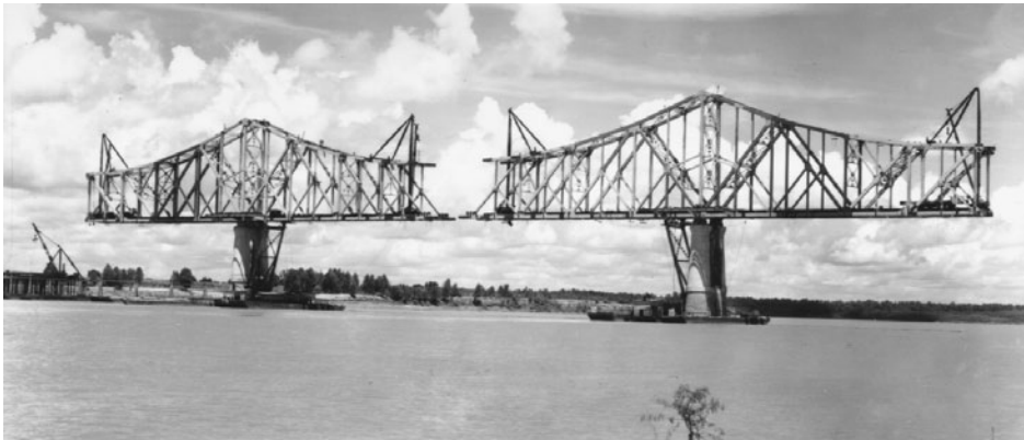
FIGURE 1.23 Balanced-cantilever erection, Governor O.K. Allen railway/highway cantilever bridge, Baton Rouge, La., 1939. First use of long balanced-cantilever erection procedure in the U.S. On each pier 650 ft (198 m) of steelwork, about 4000 tons, was balanced on the 40 ft (12 m) base formed by a sloping falsework bent. The compression load at the top of the falsework bent was measured at frequent intervals and adjusted by positioning a counterweight car running at bottom-chord level. The main spans are 848-650-848 ft (258-198-258 m); 650 ft span shown. (Courtesy of Bethlehem Steel Corporation.)
