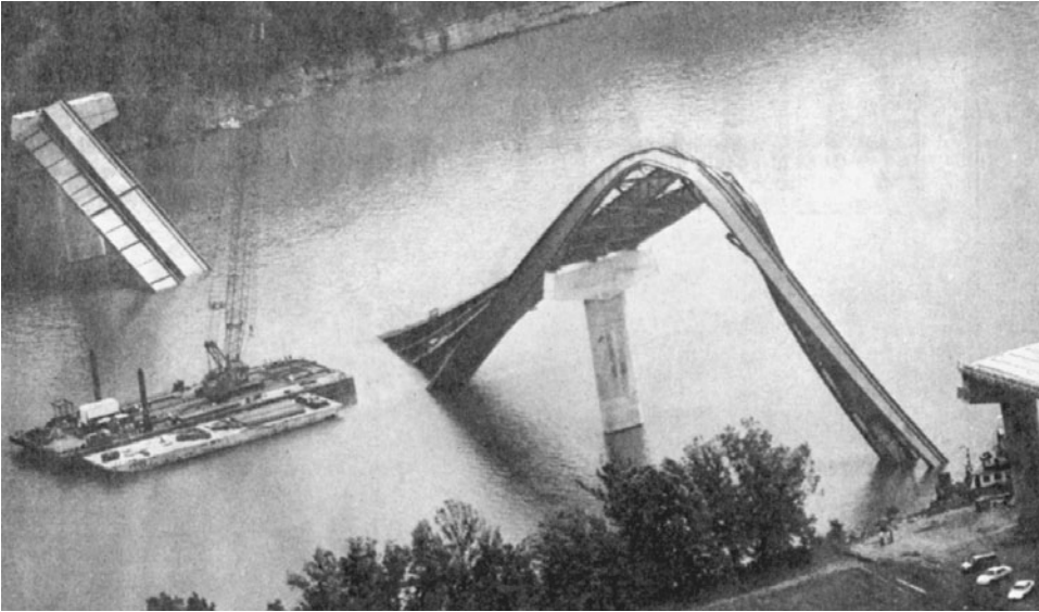
FIGURE 1.1 Failure of a steel girder bridge during erection, 1995. Steel bridge failures such as this one invite suspicion that the construction engineering aspects were not properly attended to.
