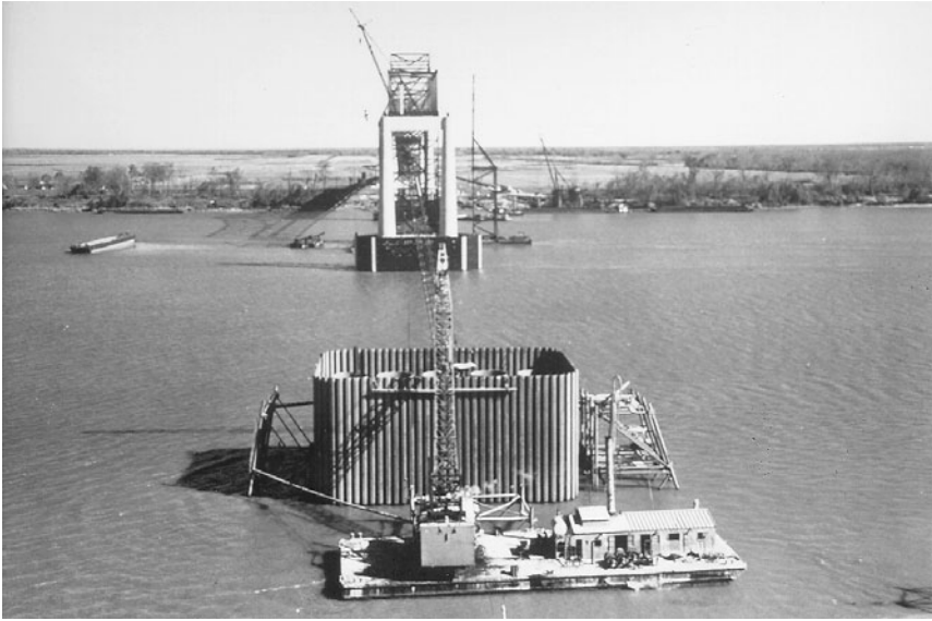
FIGURE 3.15 Open-caisson positioned within steel jackets on “pens.”
