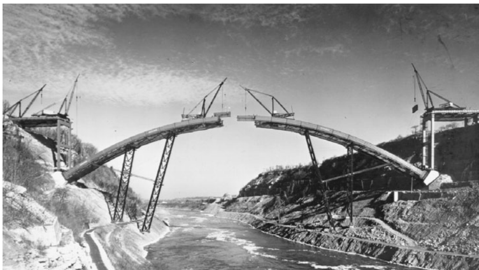
FIGURE 1.4 Lewiston-Queenston arch bridge, near Niagara Falls, New York, 1962. The longest fixed-arch span in the U.S. at 1000 ft (305 m); rise is 159 ft (48 m). Box arch-rib sections are typically about 3 \times 13\text{-}1/2 ft ( 0.9 \times 4.1 m) in cross-section and about 44\text{-}1/2 ft (13.6 m) long. Job was estimated using erection tiebacks (same as shown in Figure 1.3 ), but subsequent studies showed the long, sloping falsework bents to be more economical (even if less secure looking). Much permanent steelwork was used in falsework bents. Derricks on approaches load steelwork onto material cars that travel up arch ribs. The 115-ton-capacity travelers are shown erecting the last full-length arch-rib sections, leaving only the short, closing crown sections to be erected. Canada is at left, the U.S. at right. (Courtesy of Bethlehem Steel Corporation.)
