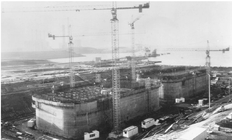
FIGURE 3.23 Large concrete box caissons fabricated in construction basin for subsequent deployment to site by self-flotation, Great Belt Eastern Bridge, Denmark.
