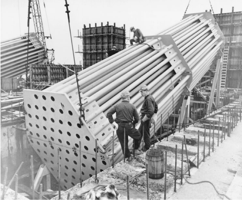
FIGURE 1.38 Pipe-type anchorage for parallel-wire-strand (PWS) cables, Newport Bridge suspension spans, Narragansett Bay, R.I., 1967. Pipe anchorages shown will be embedded in anchorage concrete. Socketed end of each PWS is pulled down its pipe from upper end, then seated and shim-adjusted against heavy bearing plate at lower end. Pipe-type anchorage is much simpler and less costly than standard anchor-bar type used with aerial-spun parallel-wire cables (see Figure 1.25B ). (Courtesy of Bethlehem Steel Corporation.)
