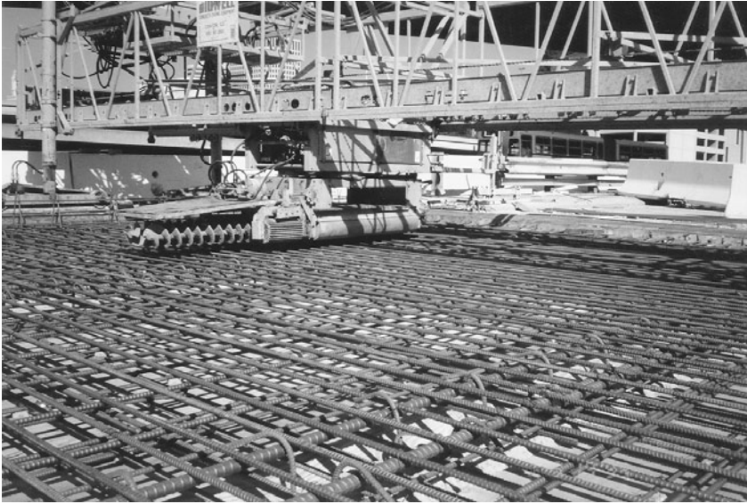
FIGURE 4.5 Bridge deck reinforcement with bidwell finishing machine.
